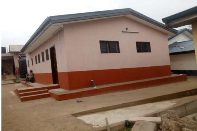
CONSTRUCTION OF 10 SEATER WC AT ADABRAKA CLUSTER OF SCHOOLS
