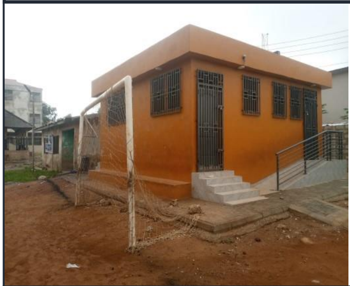
CONSTRUCTION OF 6 SEATER WC AT LIBERTY AVENUE CLUSTER OF SCHOOLS
