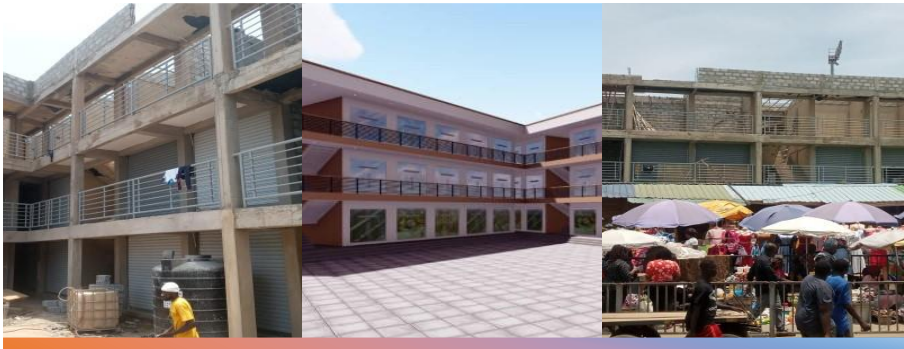
CONSTRUCTION OF 1 NO. 64 UNIT LOCABLE SHOPS AT TEMA STATION
