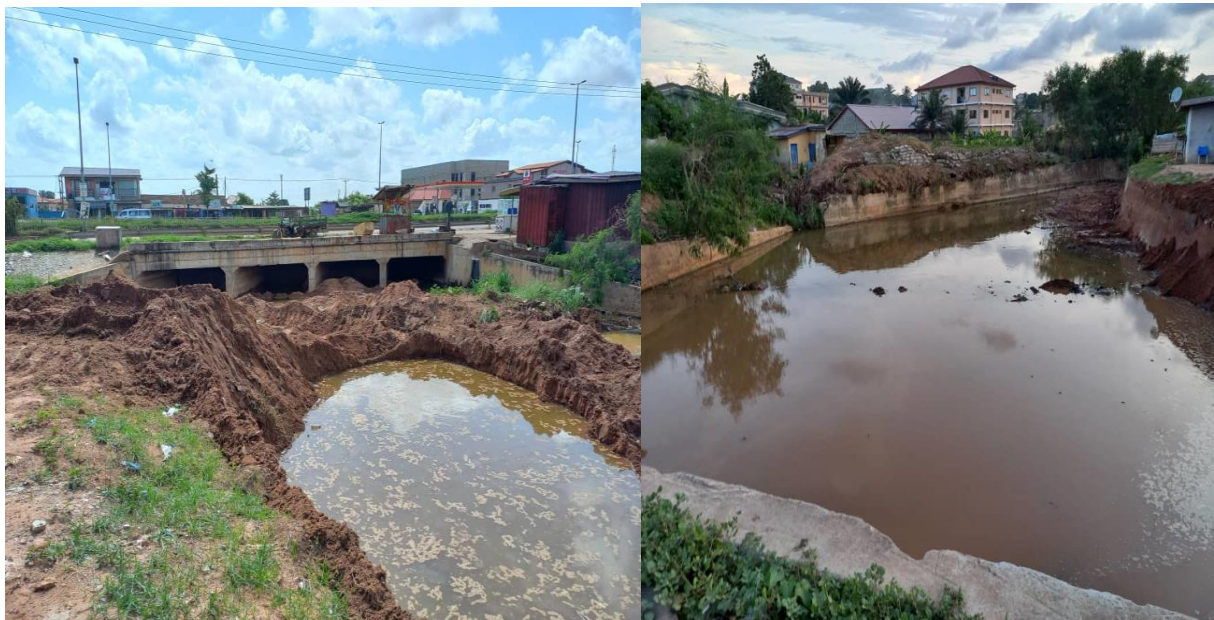
Picture 10: Desilting of Palas Town Drain
