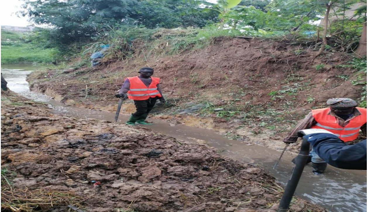
Desilted Earth Channels at Roman Ridge Police Station (450m)
