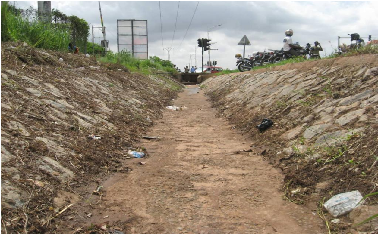
Desilting of buried and open drains at Okponglo (400m)
