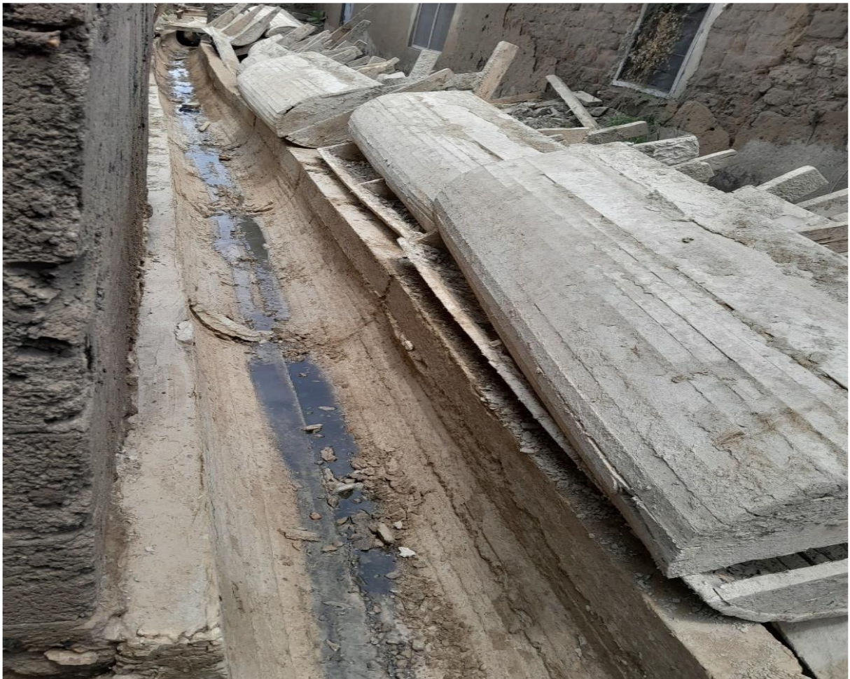
CONSTRUCTED A 0.6 M U-DRAIN
