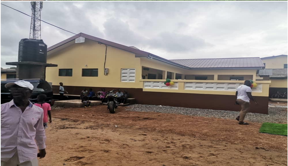
CONSTRUCTED 2-UNIT KG BLOCK WITH ANCILLARY FACILITIES AT BUBUASHIE 1 BASIC SCHOOL-OKAIKOI SOUTH SUB-METRO AMA
