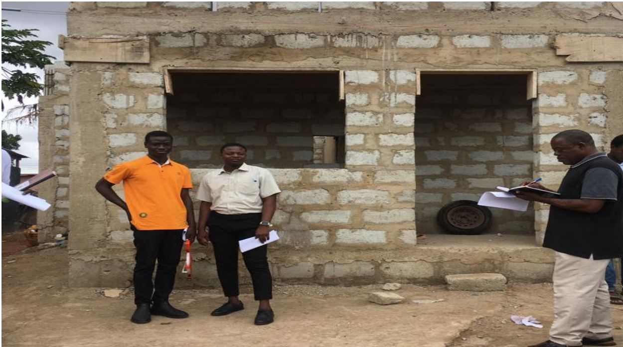
CONSTRUCTION OF 10-SEATER WC IN OKAIKOI SOUTH
