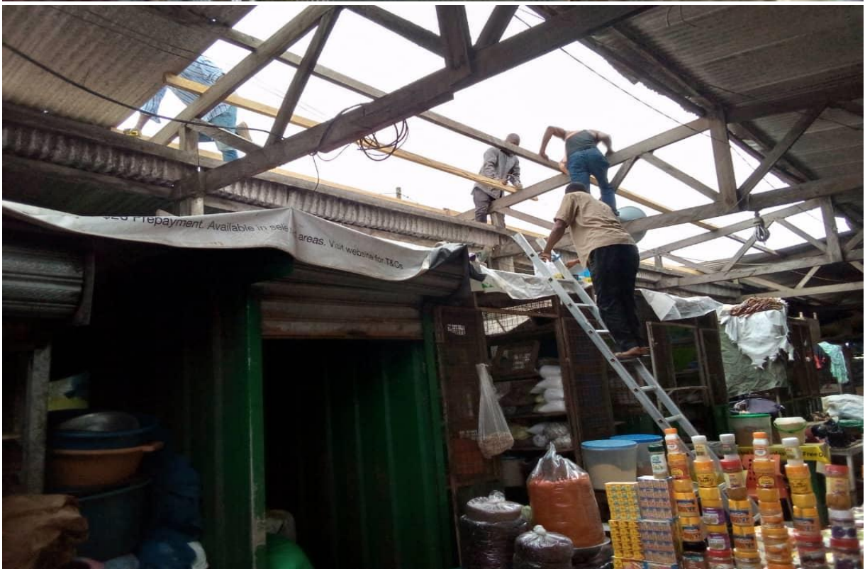
RE-ROOFING OF MAKOLA MARKET SHED RIP-OFF
