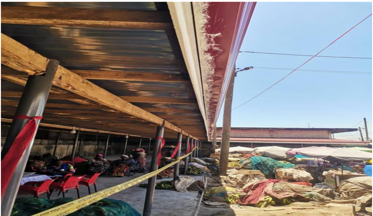
RECONSTRUCTION OF MARKET SHED AT AGBOGBLOSHIE FOR PLANTAIN SELLERS.
