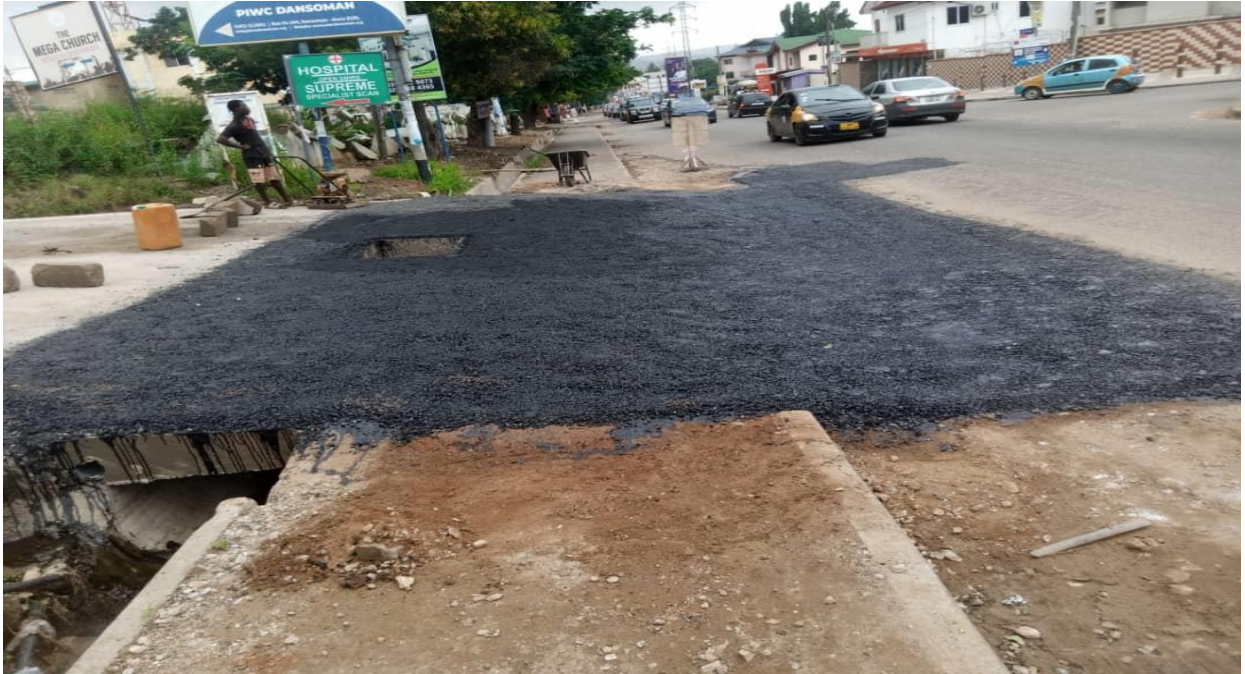
Maintenance Work at 1st Stop and Ave Maria – 100%
