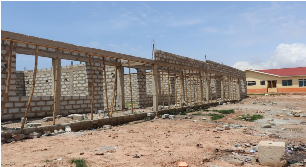
Construction of 1No. 6-Unit Classroom Block @ AME Zion School, Nasarawa. – 55%
