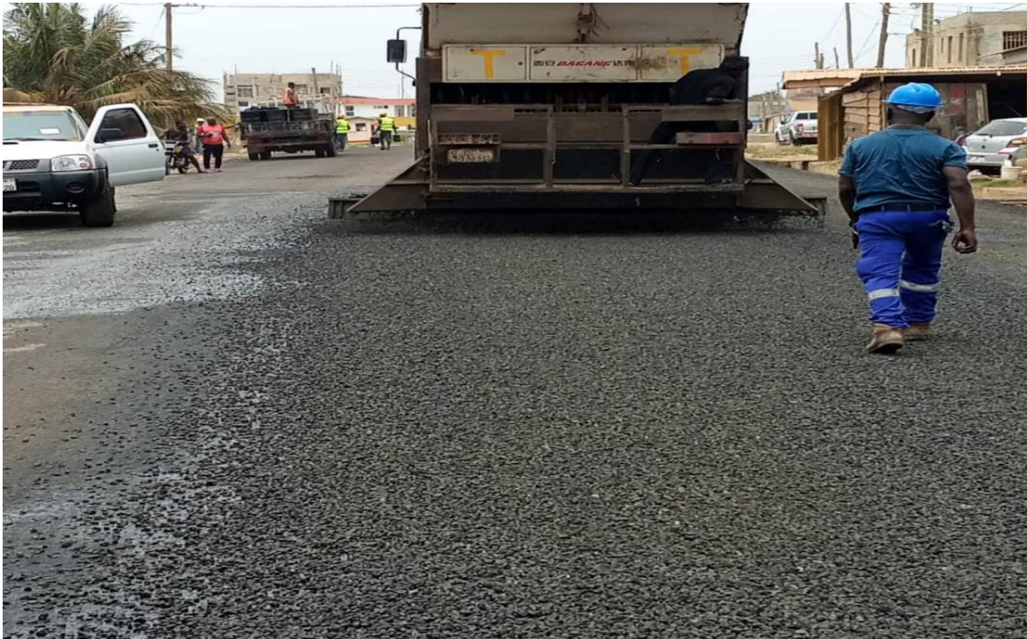
Surfacing of Manye Addokailey Street and Others – 50%
