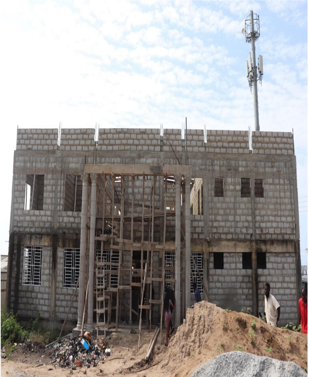
Completion of 30 bed capacity Hospital at Gbegbeyise – 70%
