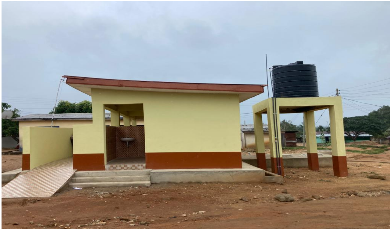
1No. 6-Seater Water Closet Toilet Facility at Asuaba constructed
