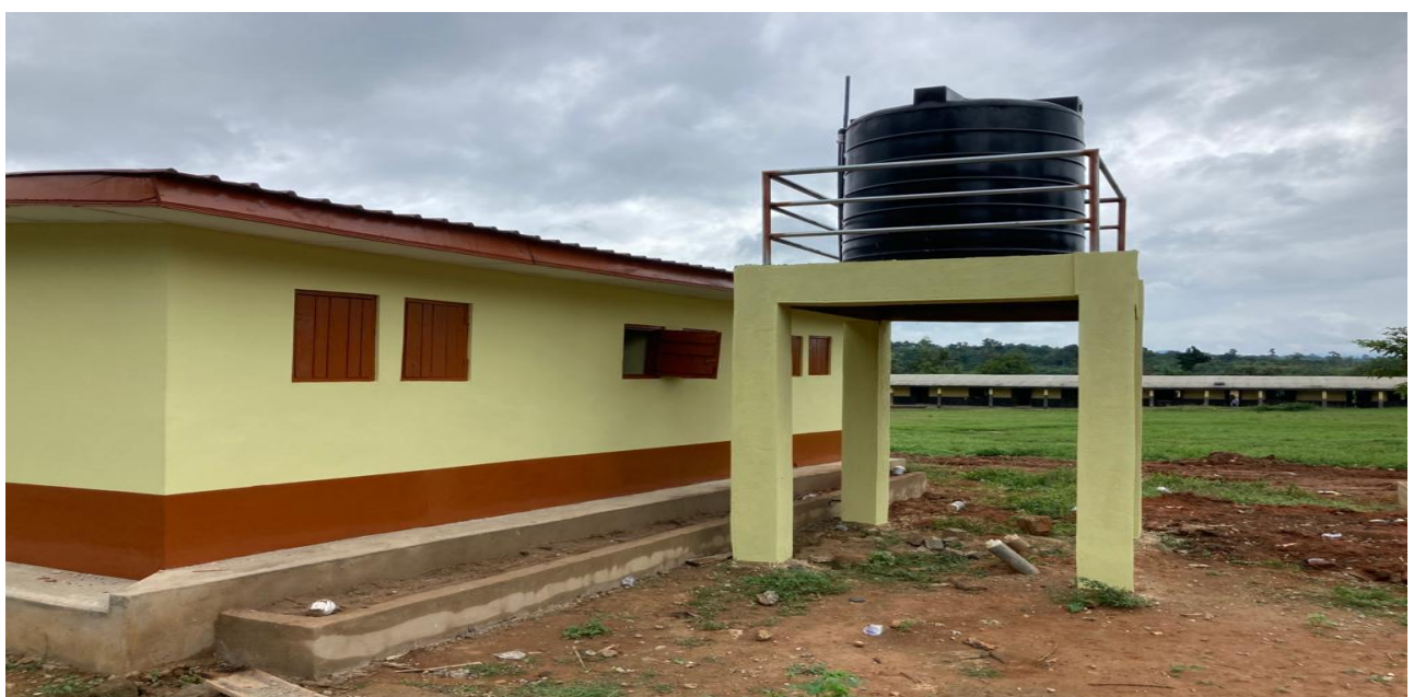
1No. 6-Seater Water Closet Toilet Facility at Domponiase constructed
