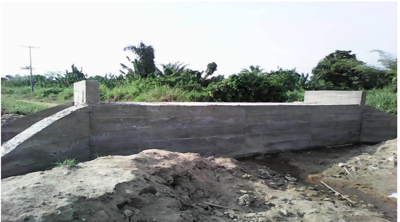
1No. 1/1200mm Diameter Pipe Culvert at Fante-Winan constructed
