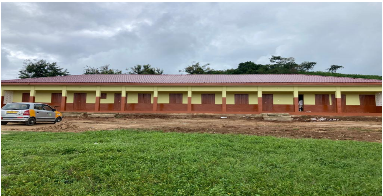
1No. 3-Unit Classroom Block with Ancillary Facilities at Domponiase constructed
