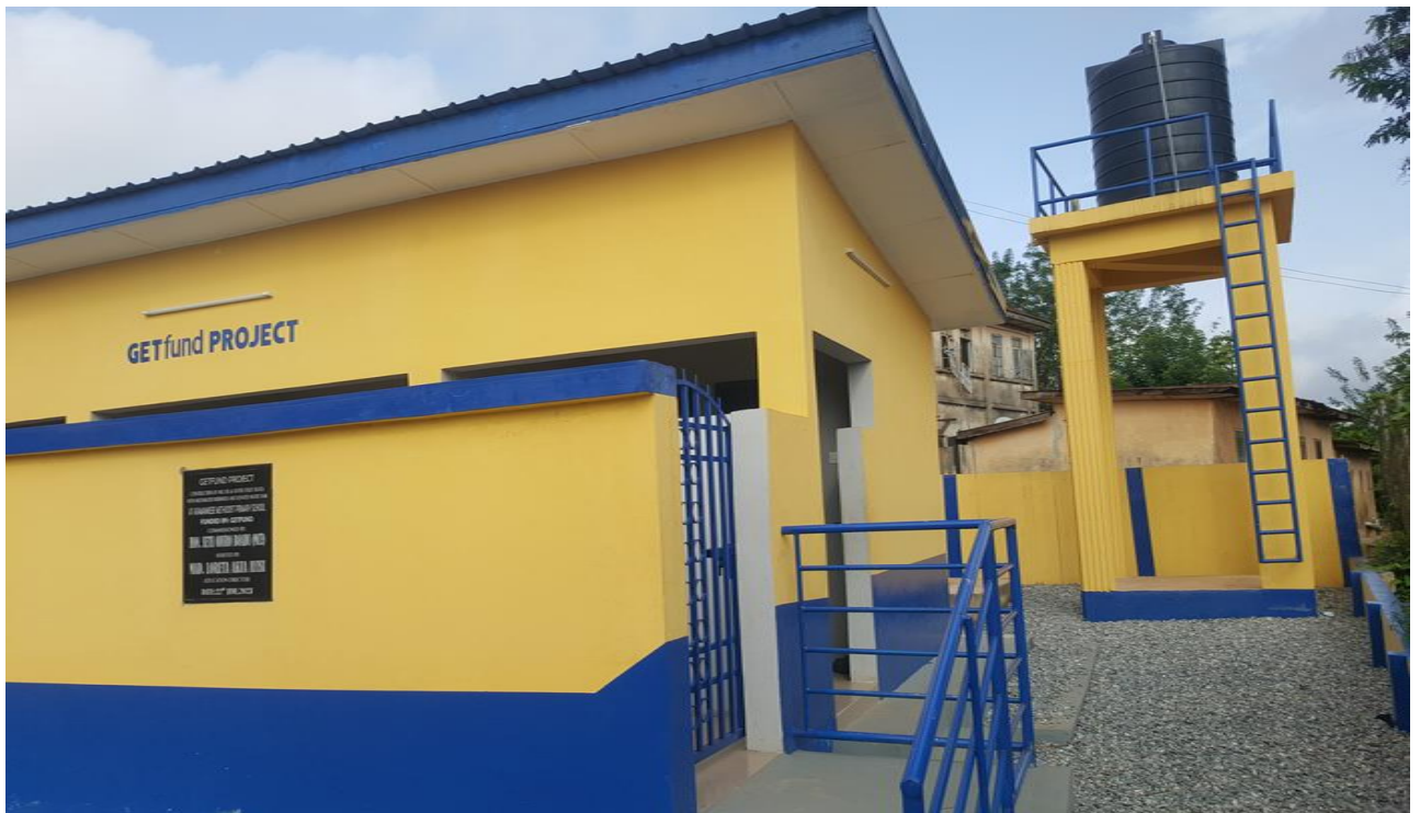
Constructed 1No. 6-Seater W/C Toilet Block with Mechanized Borehole with elevated Water Tank At Asamankese Wesley Methodist Primary School.
