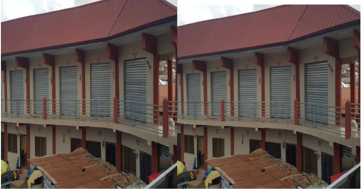
Completed the remaining 33-unit lockable store out of the 77-units at the Asamankese main lorry station.
