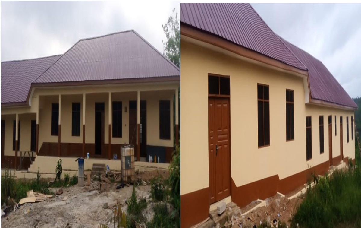
Constructed 1no. 3-unit classroom block with office store, staff common room, 2-unit urinal at Otwenkwanta.
