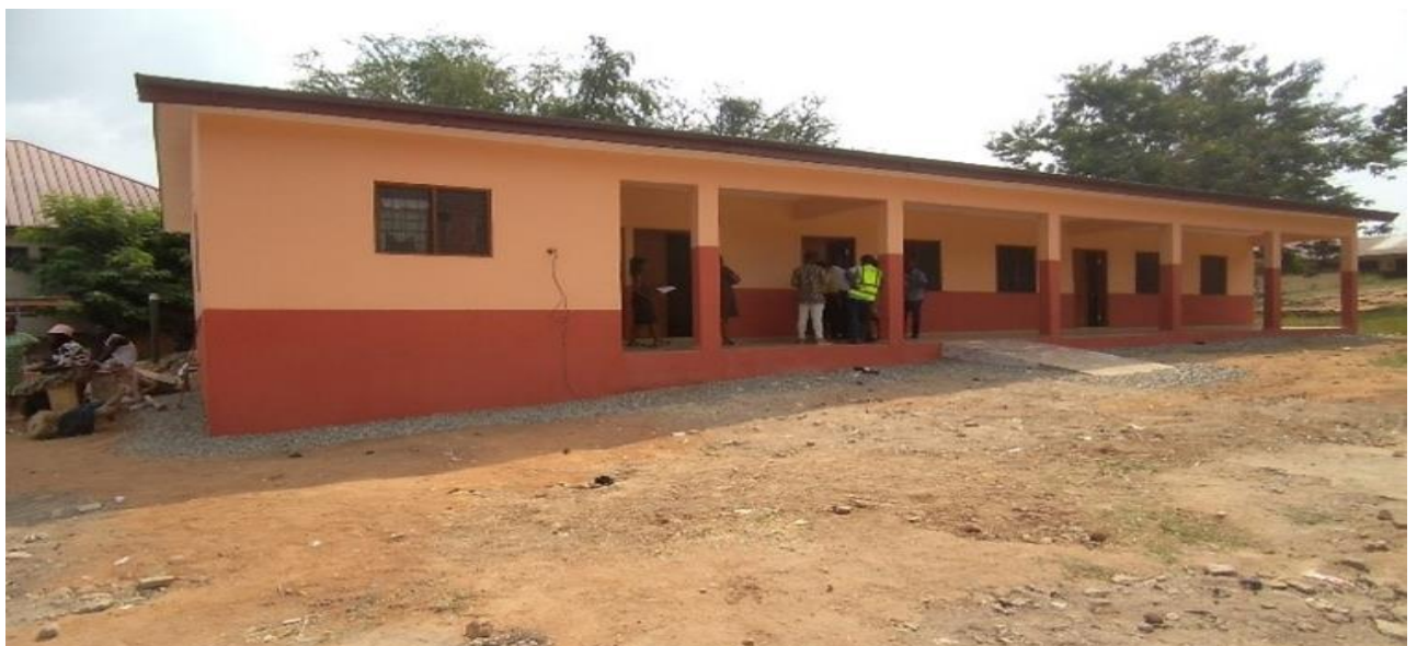
Constructed 2-unit KG block for Nana Kweku Boateng 'A' School.
