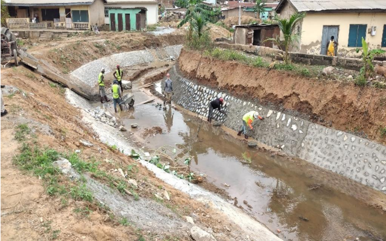
Additional works on Nsukwao Basin.
