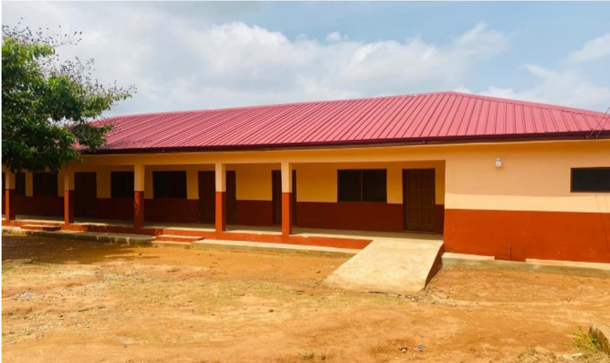
Constructed 2-unit KG block at Ada Kyeremanteng School
