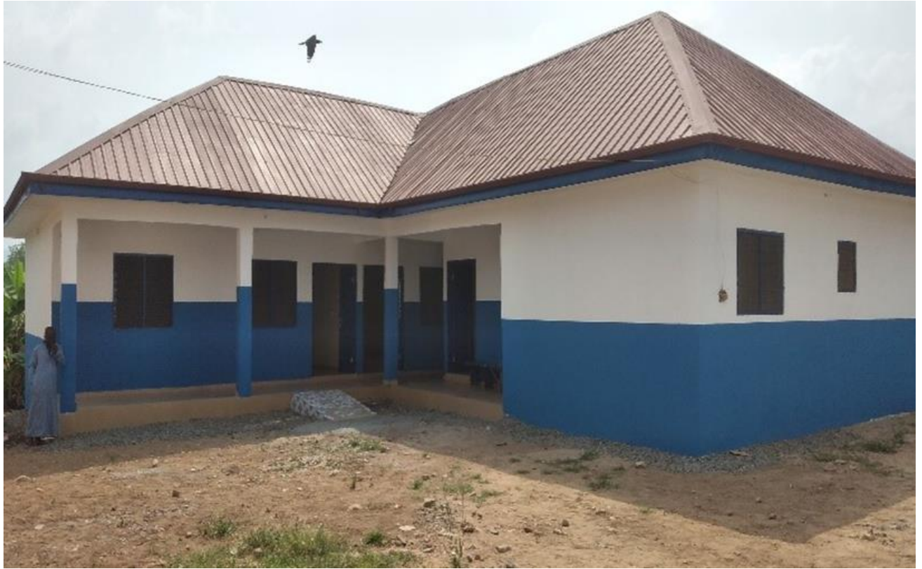
Constructed 2-unit KG block for Trinity Presbyterian Model School.
