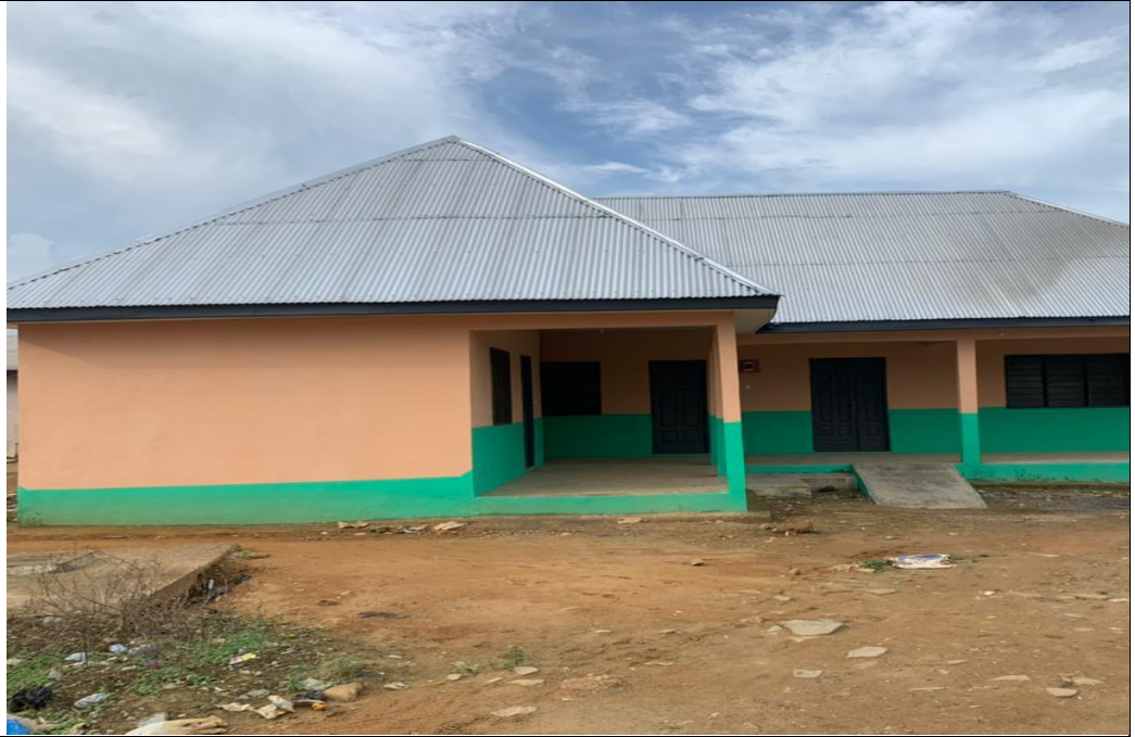
Constructed Area Council office at Akyem Akropong
