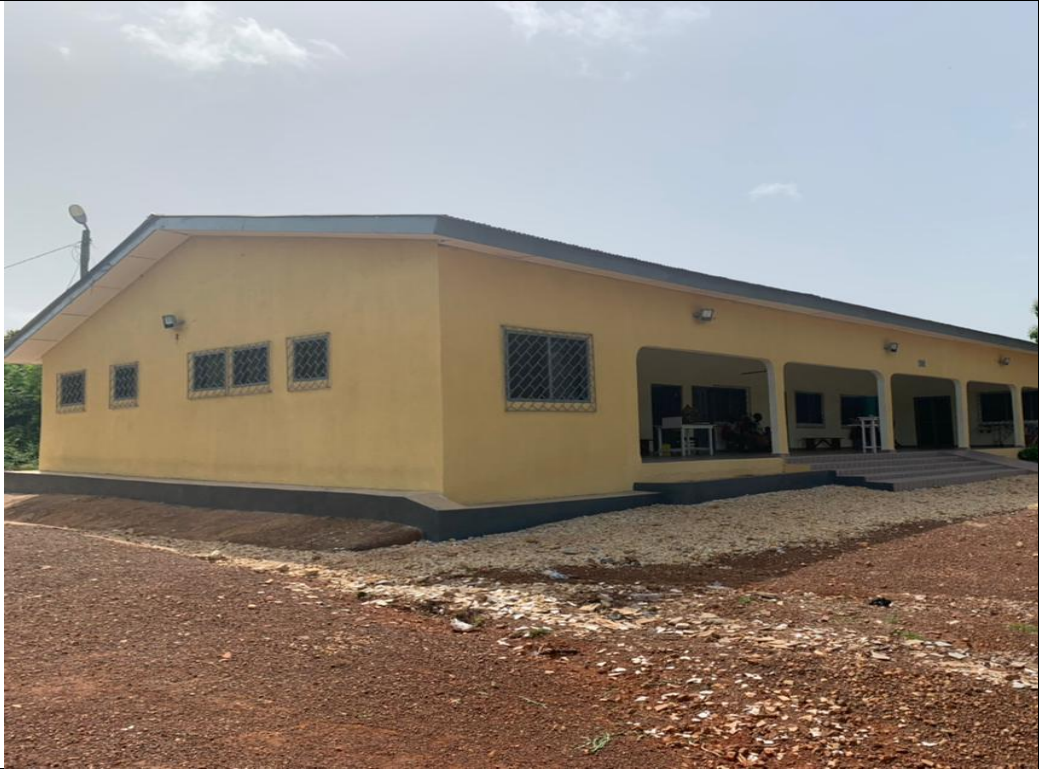
Renovated CHP's compound at Akrofufu
