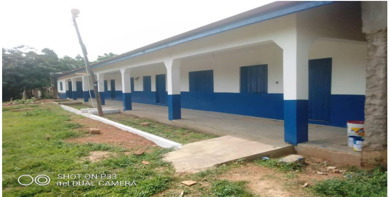
CONSTRUCTION 1 NO. 3 UNIT CLASSROOM BLOCK AT GYAKITI-DACF/RFG
