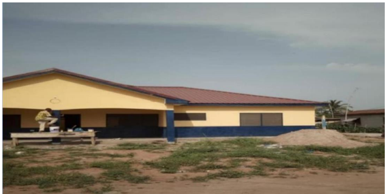
CONSTRUCTION OF POLICE STATION AT ASIKUMA – DACF
