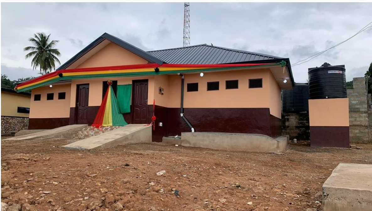
CONSTRUCTION OF 1 NO. 16-SEATER WC TOILET AT ATIMPOKU-DACF/RFG
