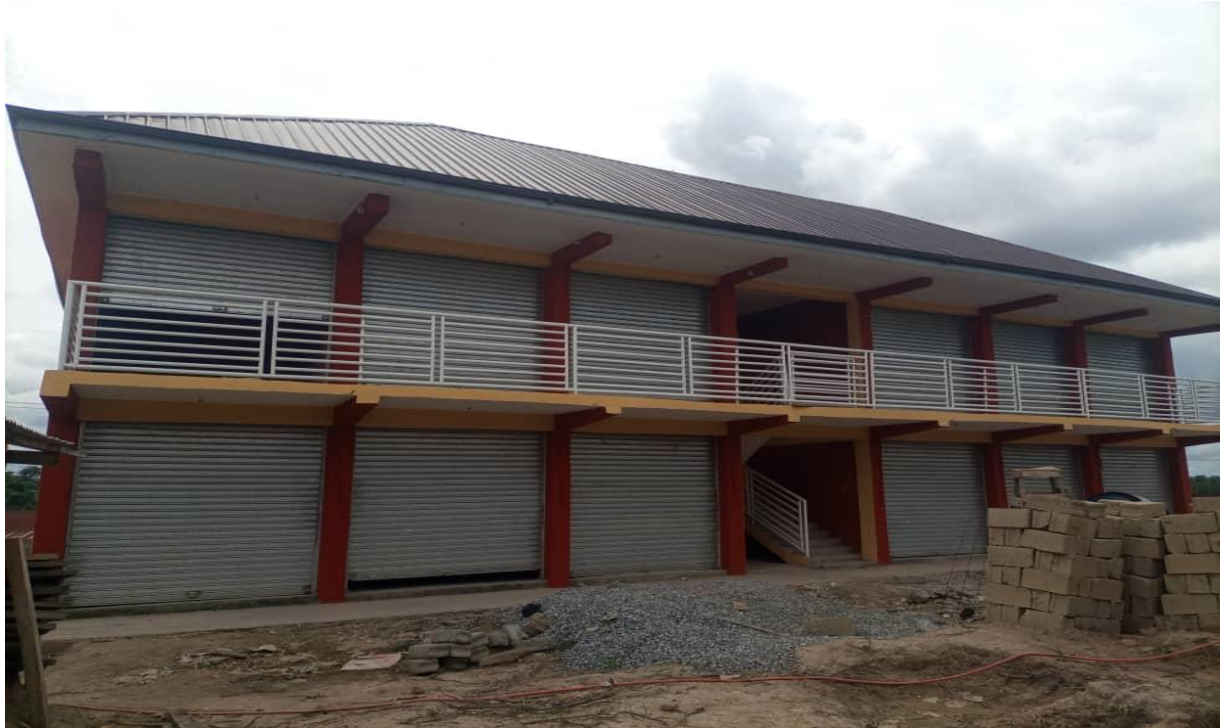
Construction of 1No. 24 lockable stores at Akim Akroso
