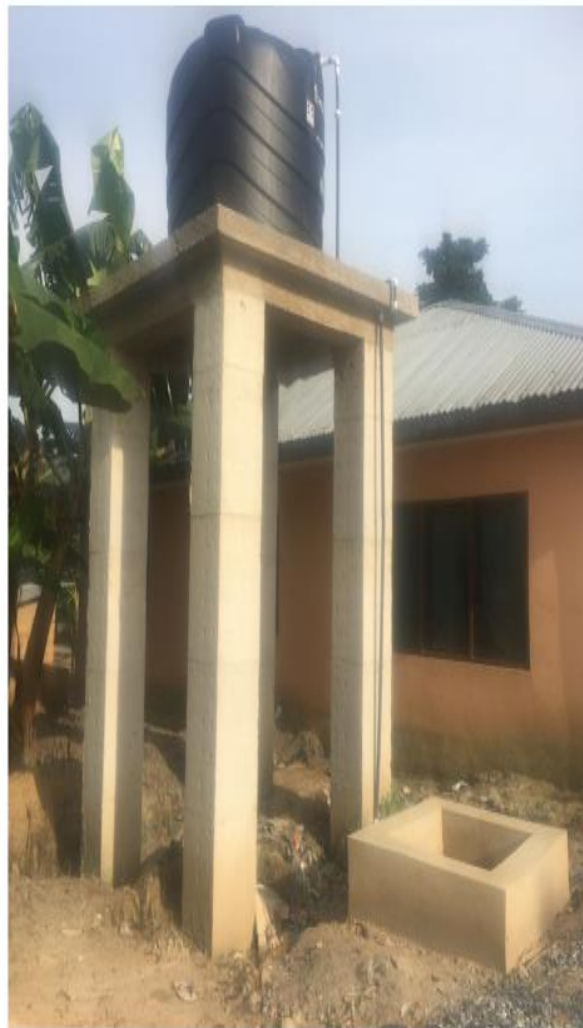
Constructed 1no. Borehole for CHPS Center at TONTRO
