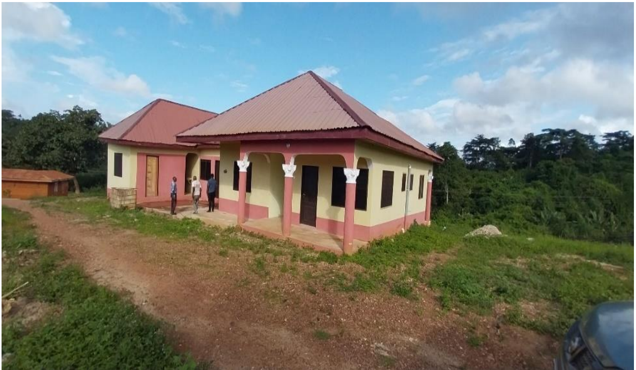
CHPS Center constructed at Besease & Aburi
