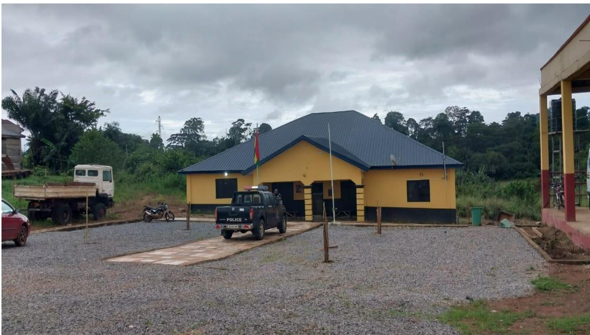
District Police Headquarters Constructed and commissioned at Diaso
