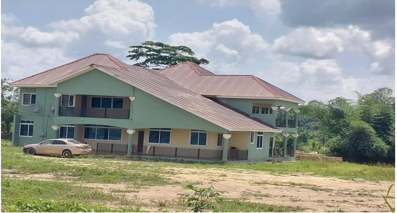
3-Bedroom Nurses Quarters constructed and in used at Diaso
