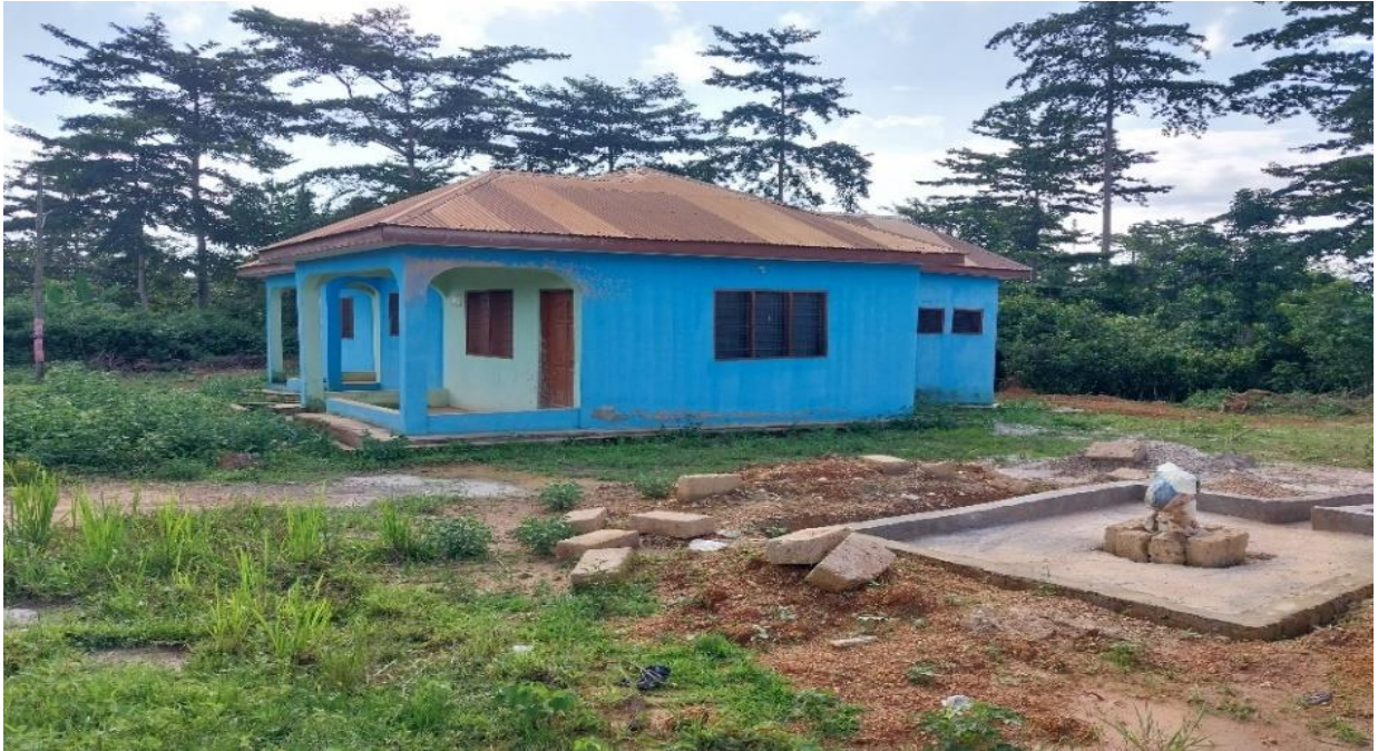
CHPS Center constructed at Anwianwia
