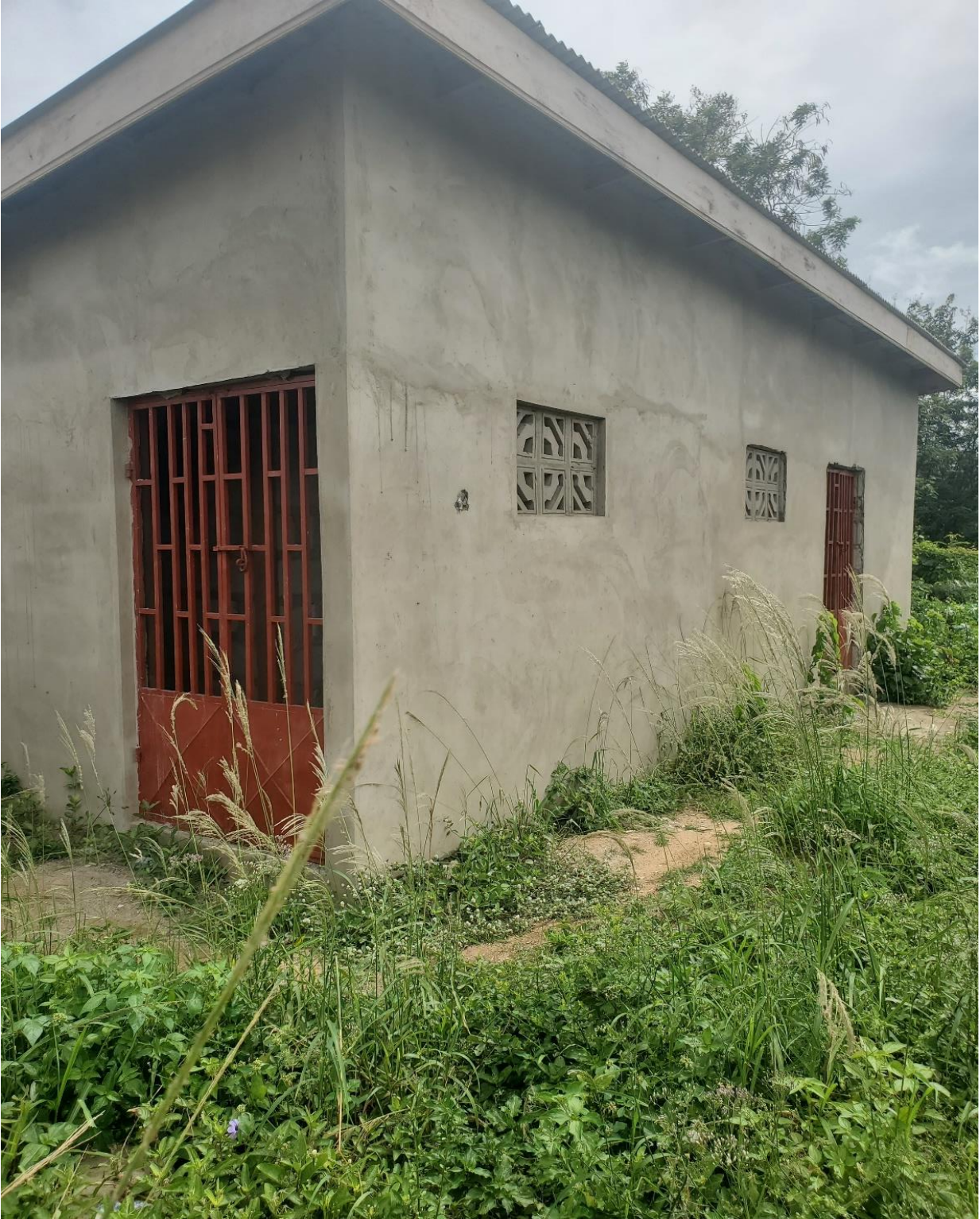
Figure 5: 1 No. 4-Seater WC & 2 No. Urinal at Elmina Junction Lorry Park
