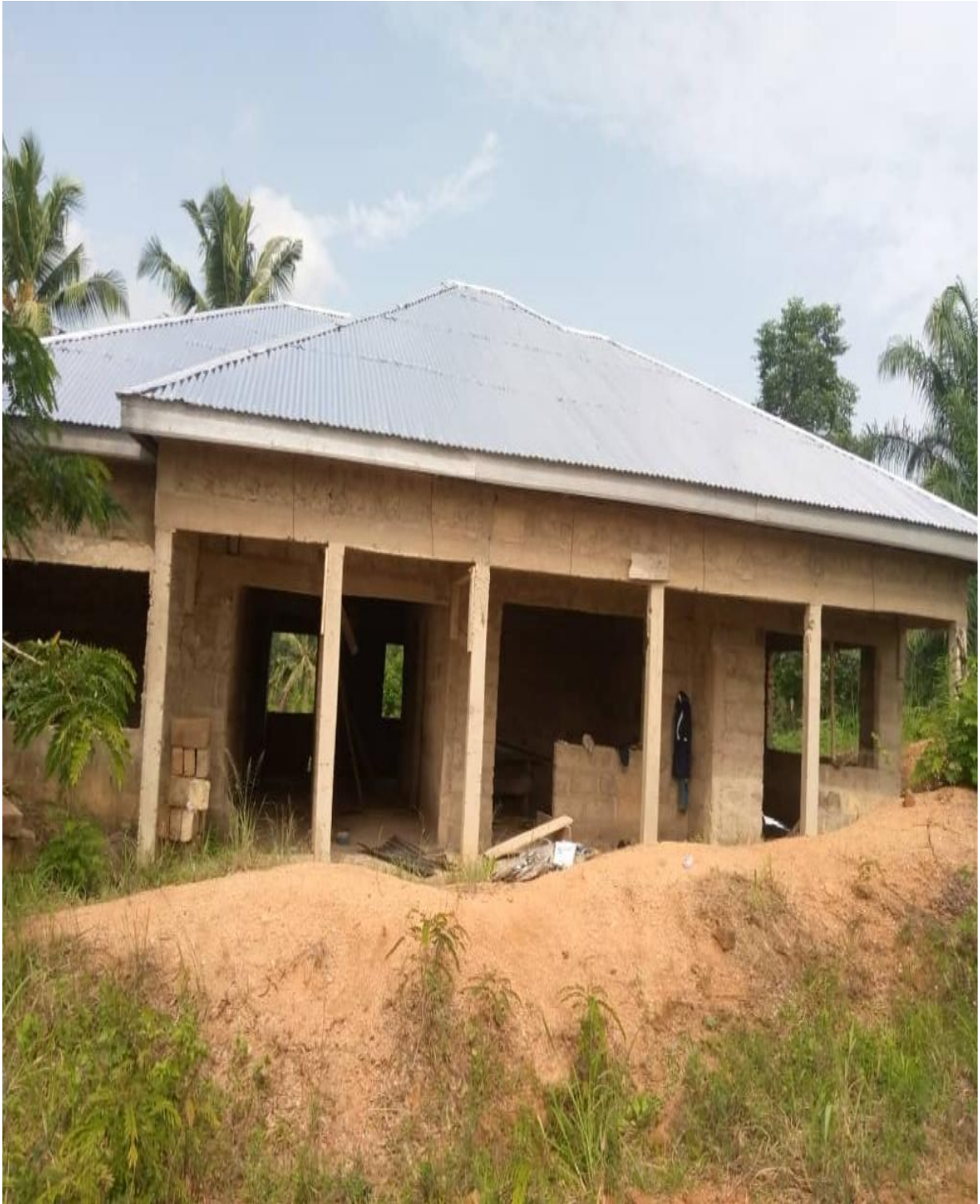
Figure 4: 1 No. CHPS Compound with Ancillary facilities at Saman, Abotar, Park (On-going)
