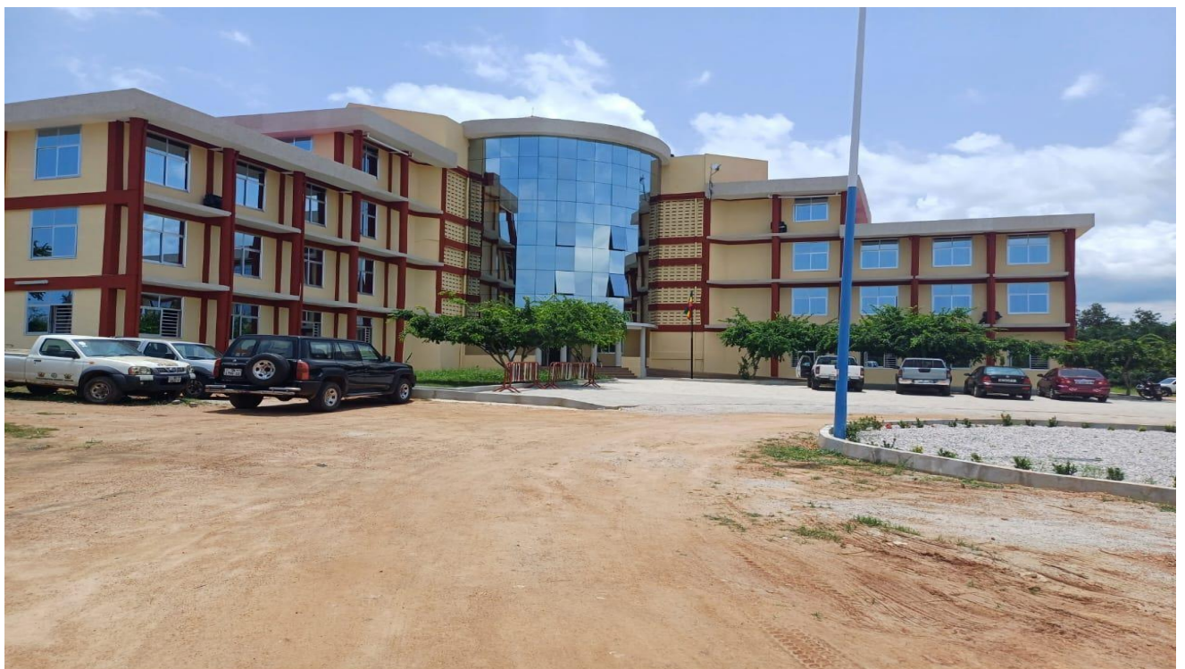
Completion of Effutu Municipal Assembly office complex
