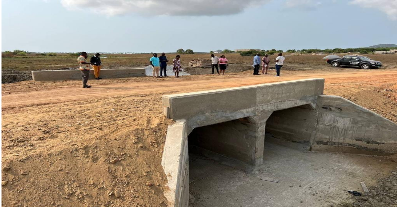
Construction of 1No. 12m (2.5m x 2.5m) Box Culvert at Ntakorfam
