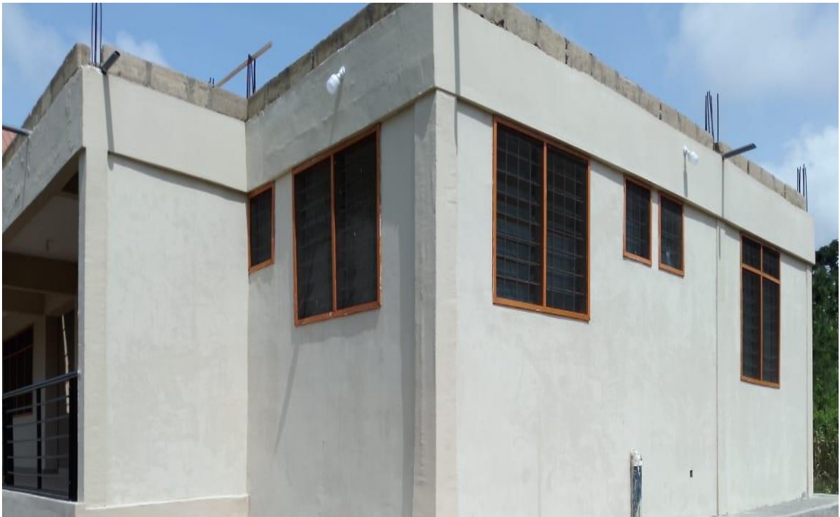
Construction of Police Station at Sewin - (Lintel Stage)
