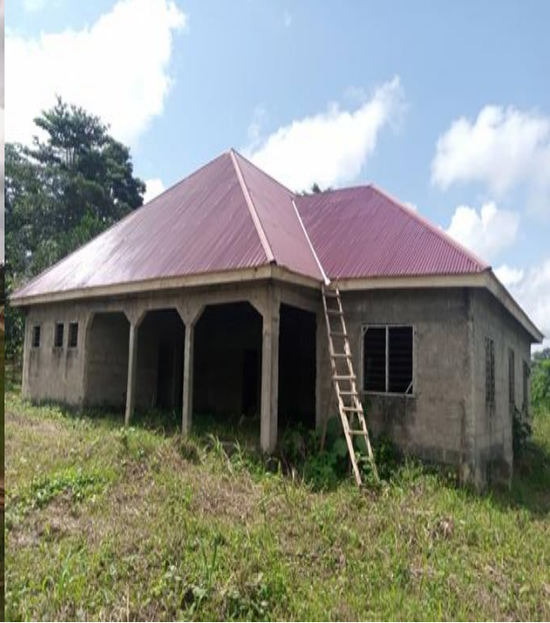
Const. of 1no. CHP Compound at Achiano W.I.P
