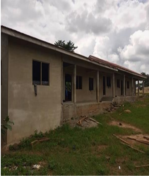
Const. of 3-units JHS classroom blk at W.I.P Dwendaama
