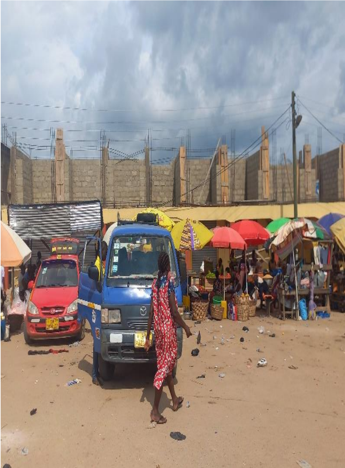
1 No. 7 Unit Trading Store at Asikuma Station Ph.II (Lintel level) IGF
