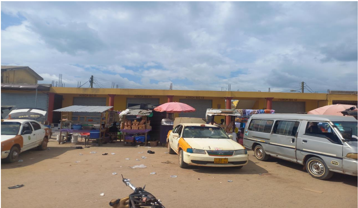
1 No. 8 Unit Stores at Asikuma Lorry Park Phl. completed DACF-RFG
