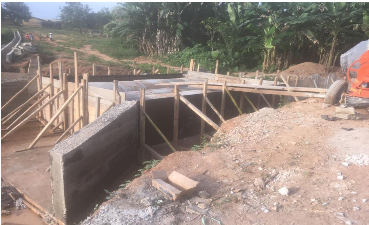
3 No. Cells Concrete Pipe Culvert & 120 Metre U-drain at Brakwa 70% completed-DACF
