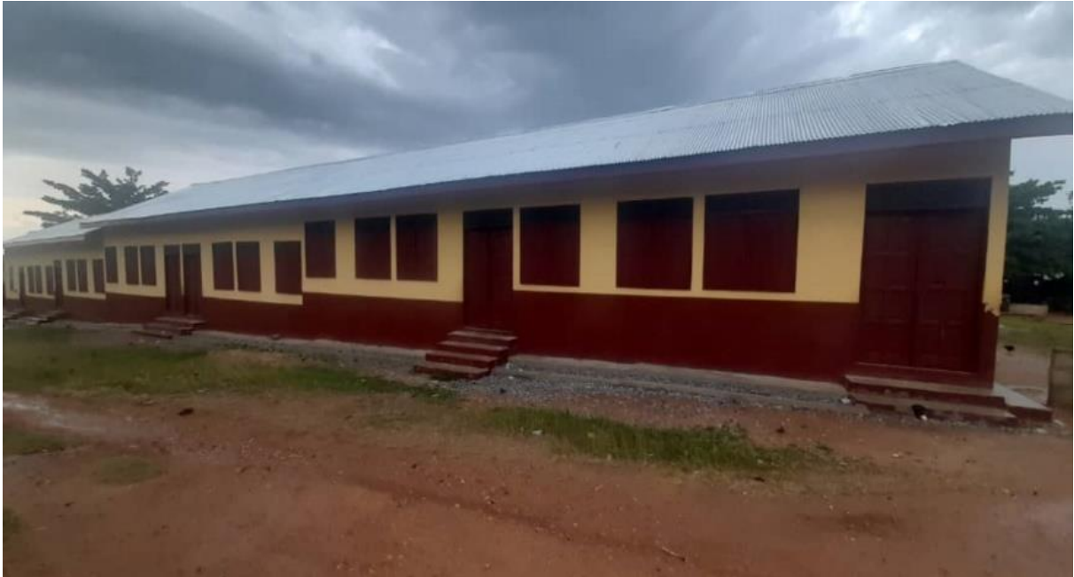
1 No. 6 Unit Classroom Block at Jamra completed DACF
