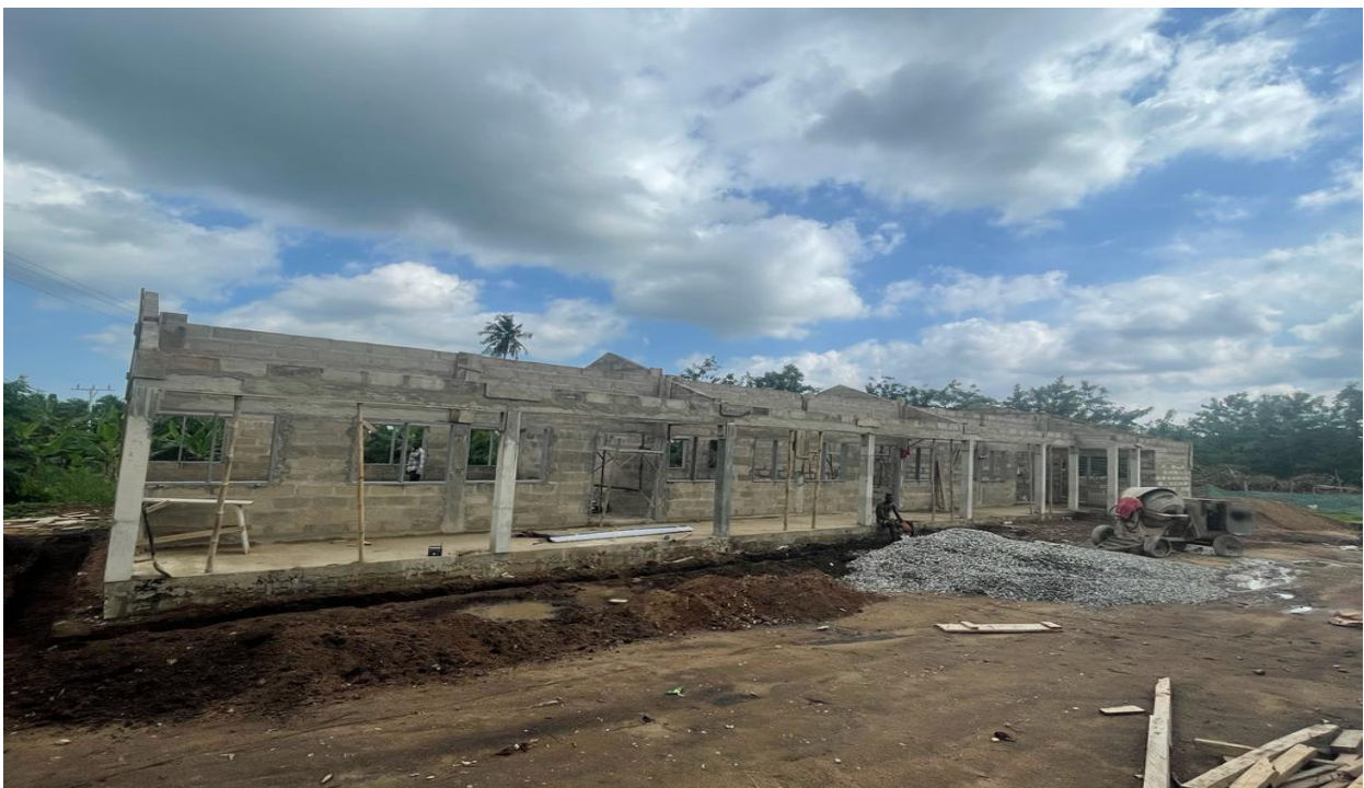
Ongoing construction of 3-unit classroom Block at Agona Nkumkum (35% completed)
