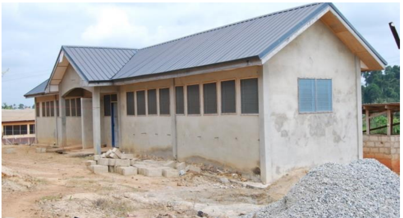
Boys Latrine at Nsaba SHS
