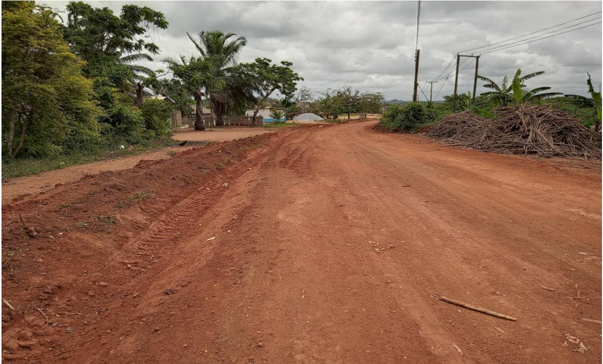
6. Reshaping of Putubiw - Apewosika Feeder Road completed.
