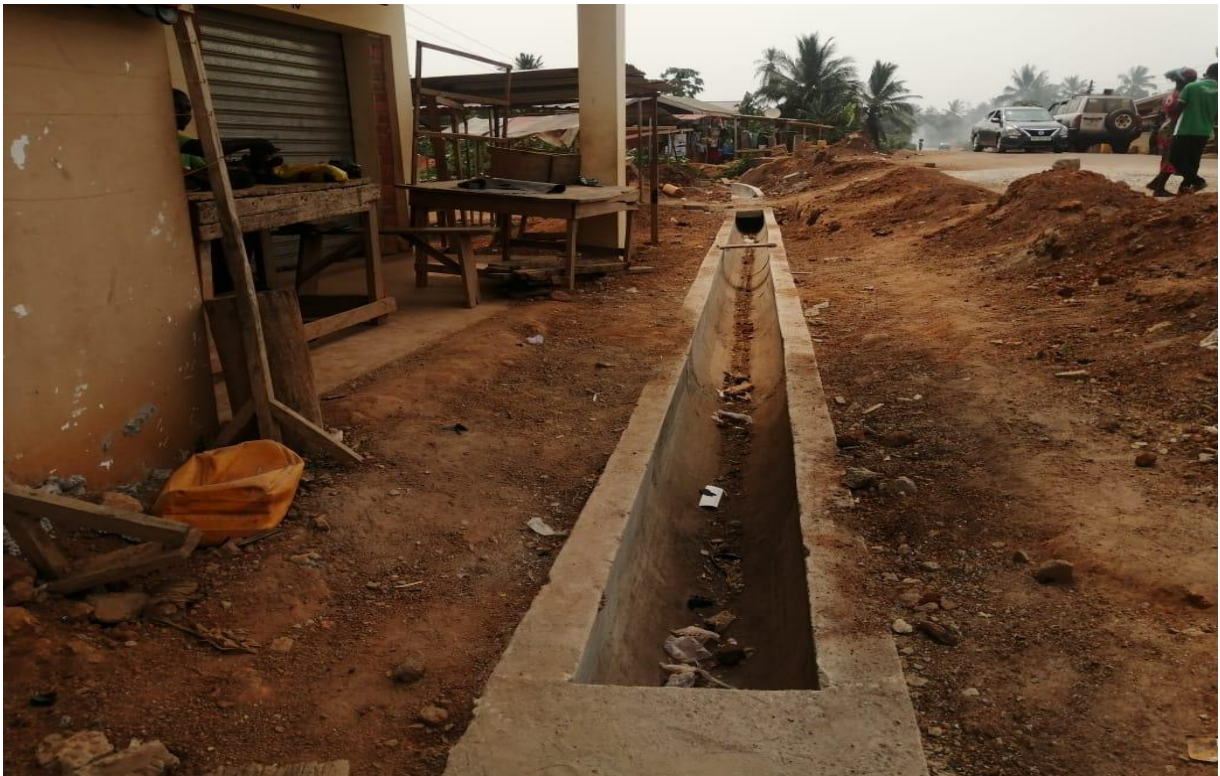
13. Construction of 249m (450mm diameter) U-drain at Asebu completed.
