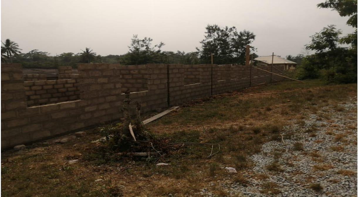
12. Construction of 1 No. 3-Unit Classroom Block at Musunkwa ongoing (50%).
