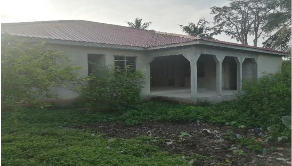
10. Completion of 1No. CHPS Compound at Abaka ongoing (51%).
