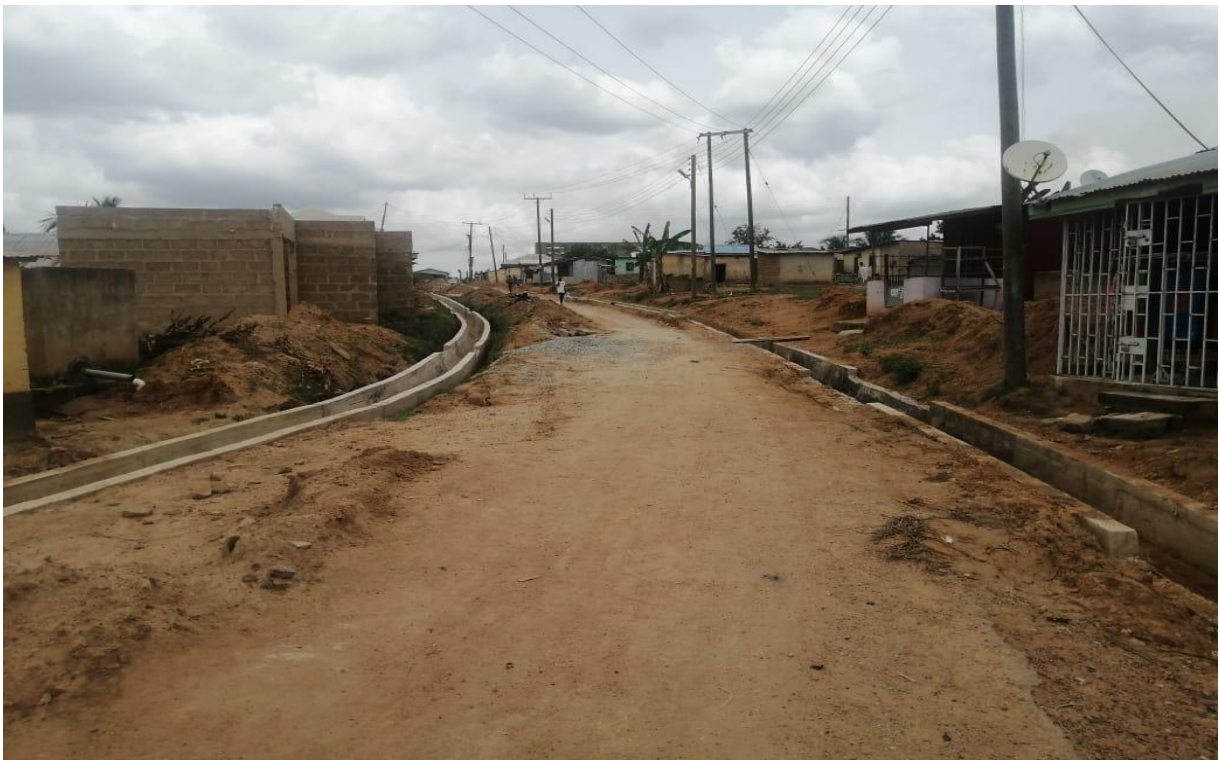
11. Construction of 406m (600mm diameter) U drain in Abura Dunkwa completed
