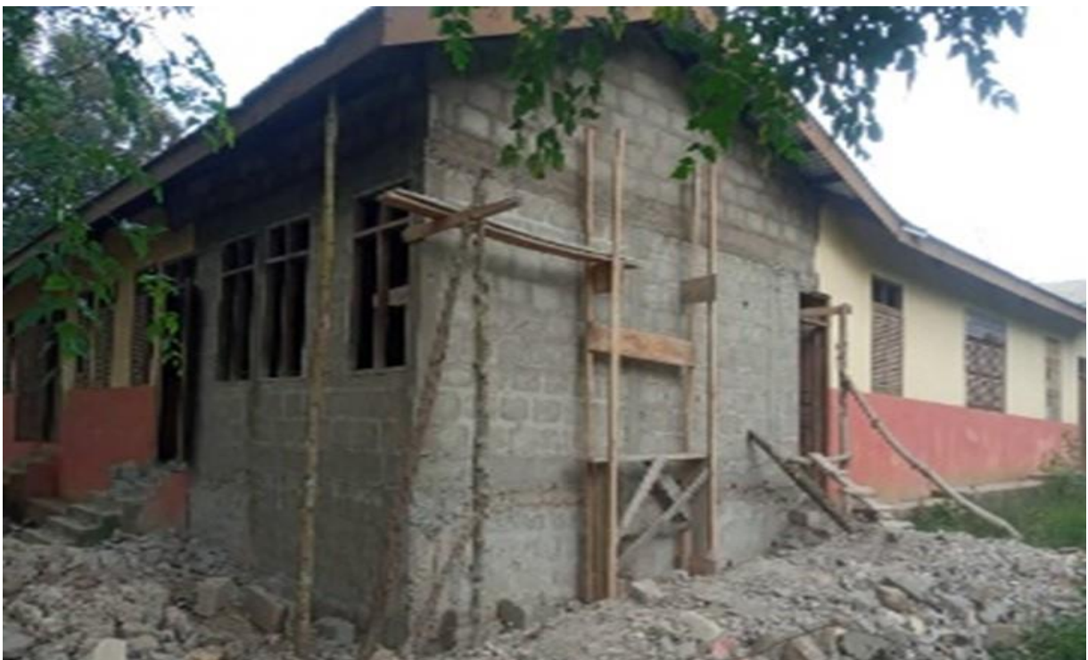
7. Rehabilitation of Ansafuna D/A Primary & KG School Block ongoing (86%).
