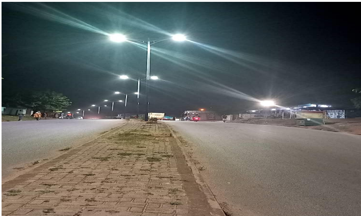
Supplied and Installed & Commissioned Streetlights at Urban Sunyani. (GSCSP)
