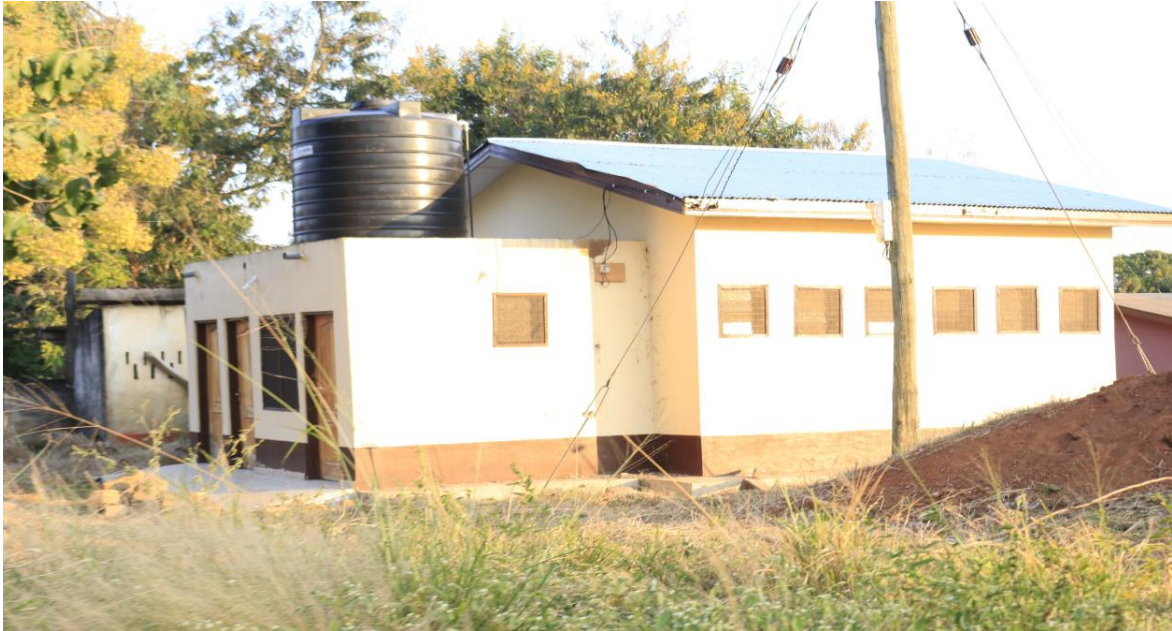
Constructed a 12-Seater Water Closet Toilet Facility at Ridge Experimental School, Sunyani Completed and in use. (DACF/RFG)
