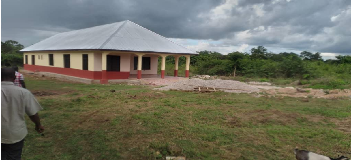
Constructed a maternity block at Goka (DACF)
