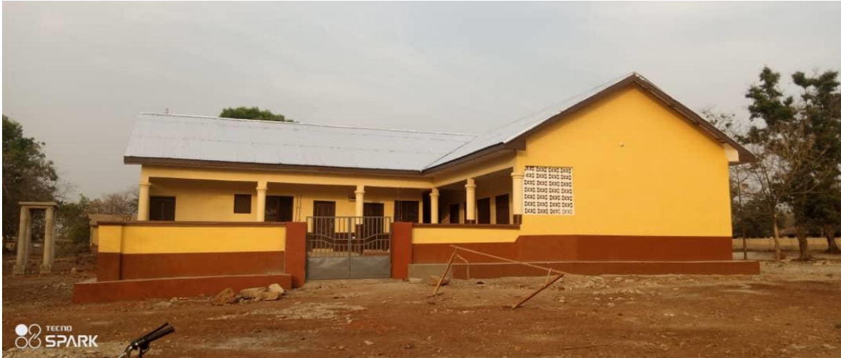
Constructed a 2-Unit KG block at Goka (DACF-RFG)
