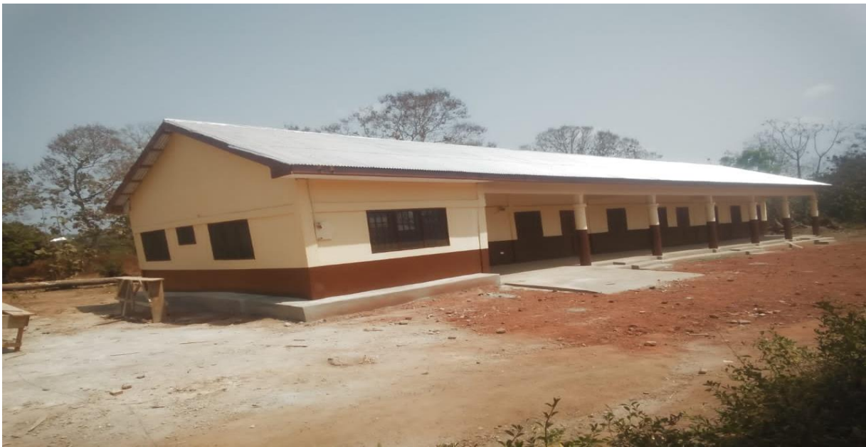
Constructed a 3 Unit Classroom Block at Nasec Presby Model (DACF-RFG)
