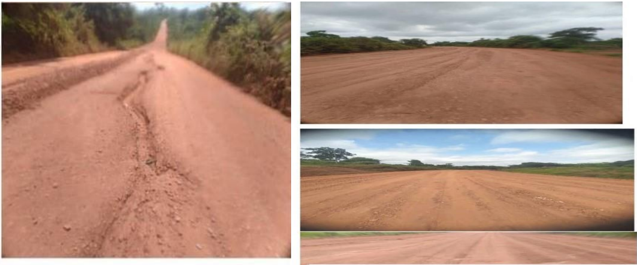
Scarified and compacted Ponkor Junction to Sampa Road (IGF)
