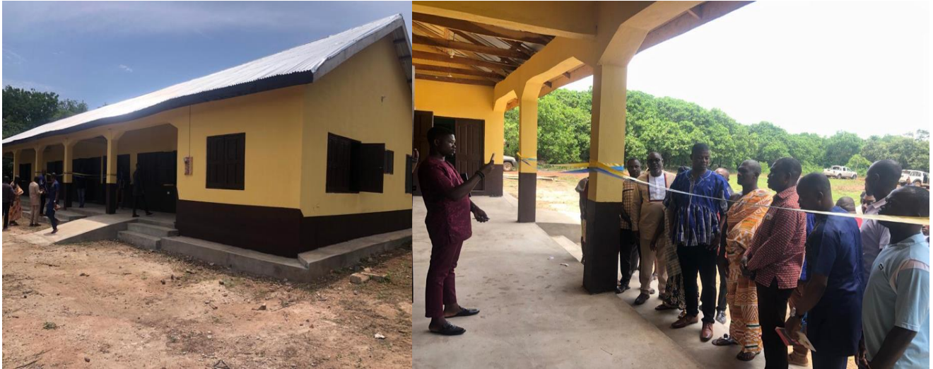
Constructed 3 Unit Classroom Block at Adinkrakrom (DAFC)
