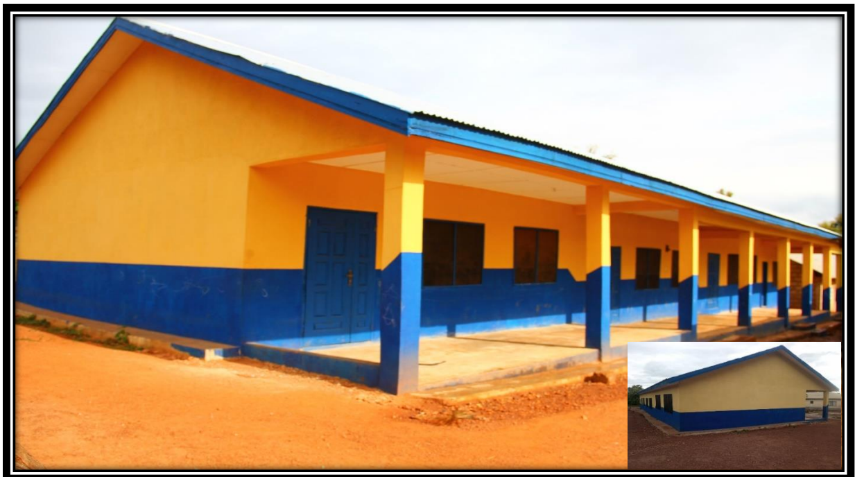
Key Achievement 4: Completed 1 No. 3-unit Classroom block for Kyeremasu SDA Primary
