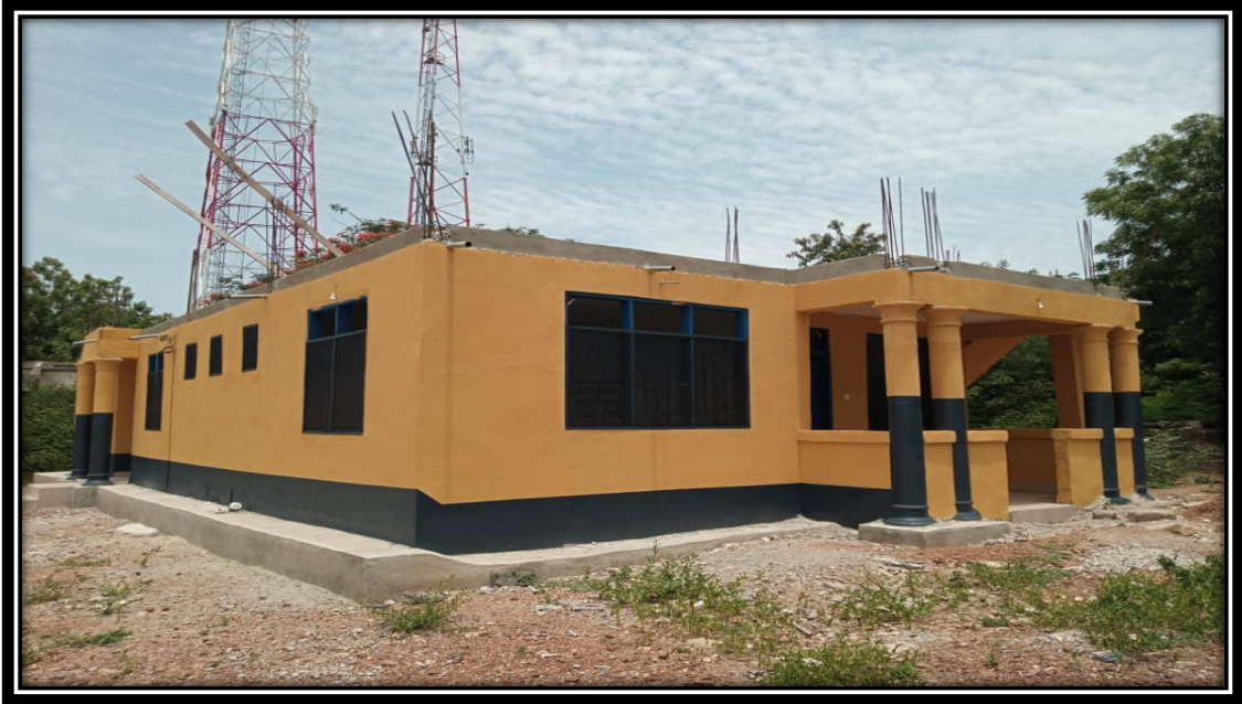
Key Achievement 1: Constructed of 1 No. Staff Accommodation for District Police Station
