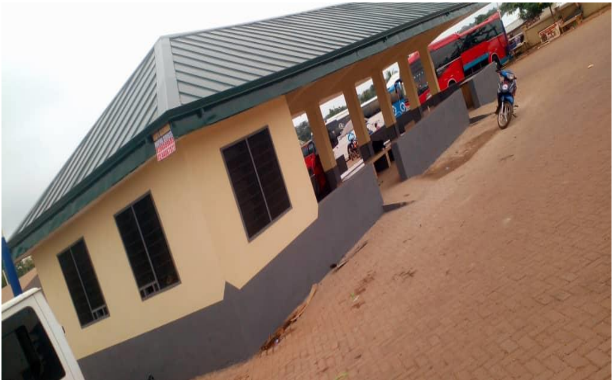
Constructed 1No waiting lounge, 1No Revenue Post and 1No. Bread sellers Shed at Dormaa Ahenkro
