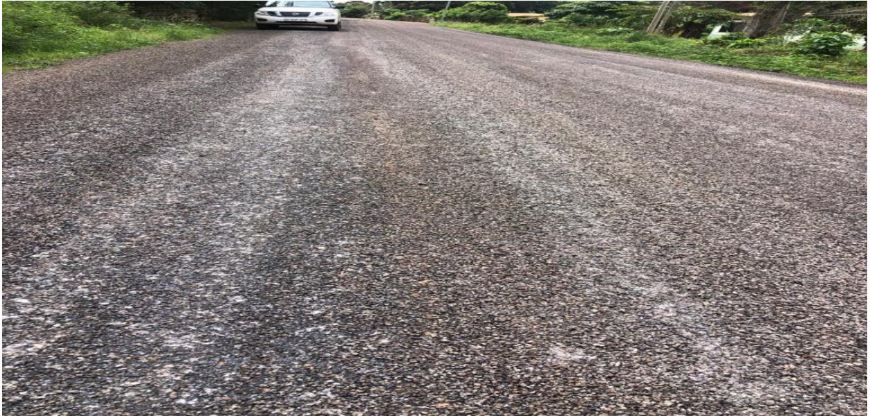
Constructed and tarred 5km town roads in Dormaa Ahenkro
