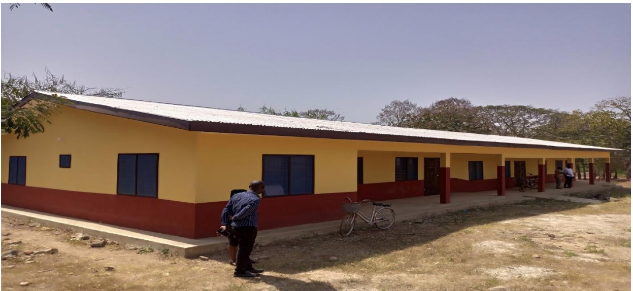
PICTURE 3: COMPLETED 1 NO. 3 UNIT CLASSROOM BLOCK AT BOTOKROM
