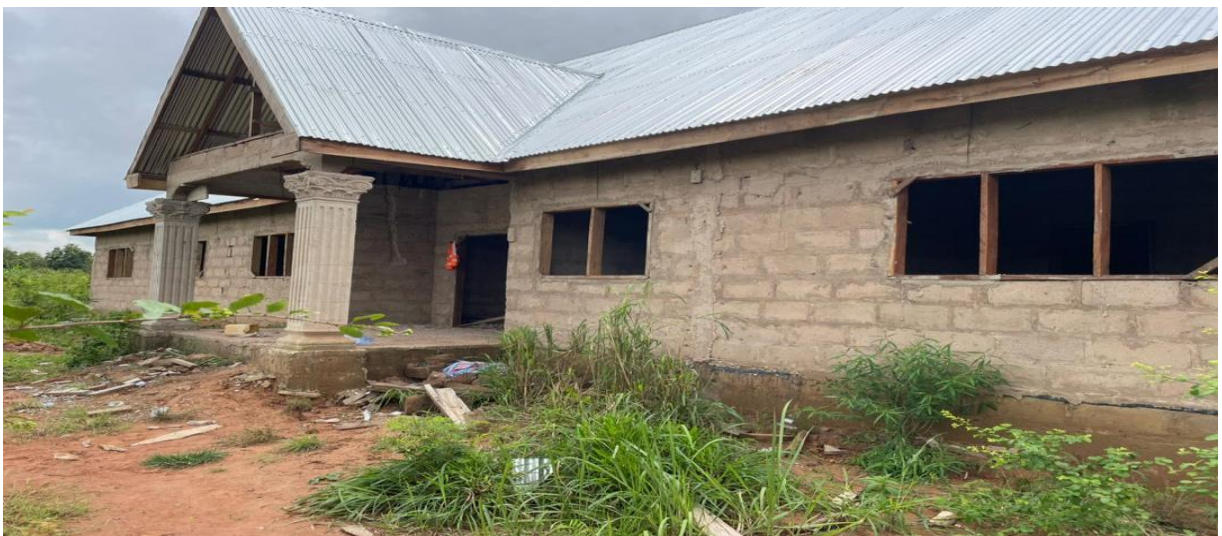
Construction of Health Directorate at Kajaji (at Roofing Stage)
