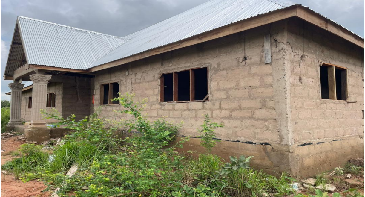
Construction of Agric Office at Kajaji (at Roofing Stage)
