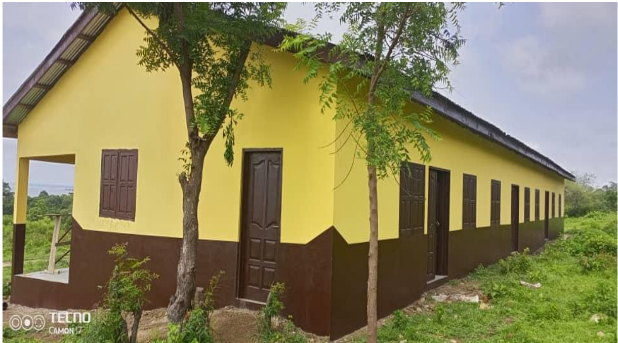
Completed 1No. 3 unit classroom block with office store at Okpalama
