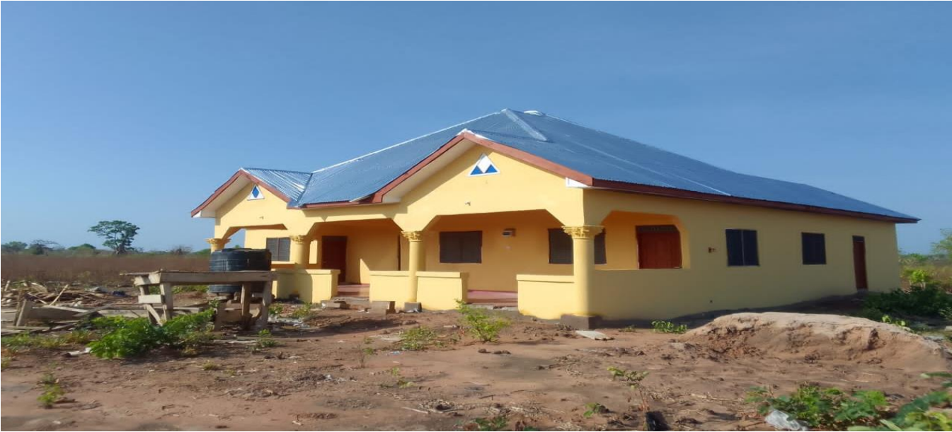
Rehabilitated 1No. 3unit classroom block at Miawani (MP)
