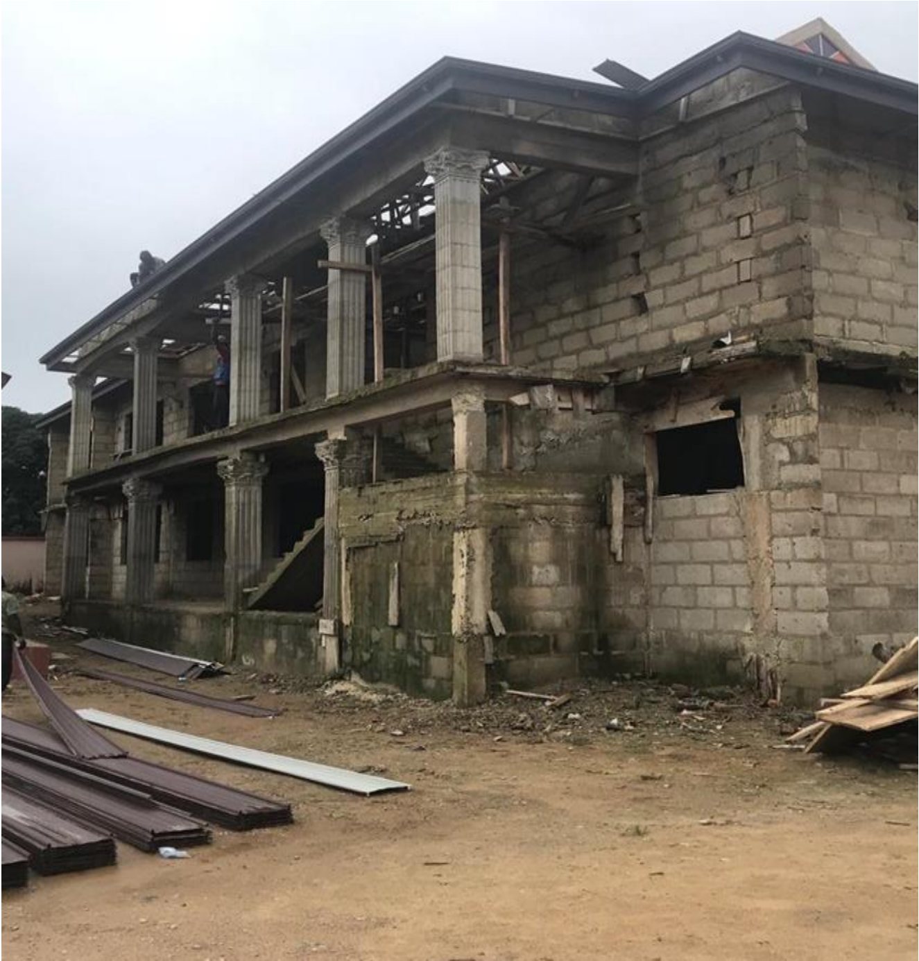
80% on-going Maternity Ward at Offinso Health Centre
