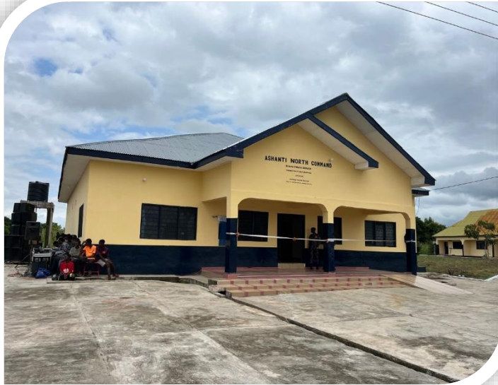
Rehabilitation of Adidwan Police Station Fund Source: IGF/DACF
