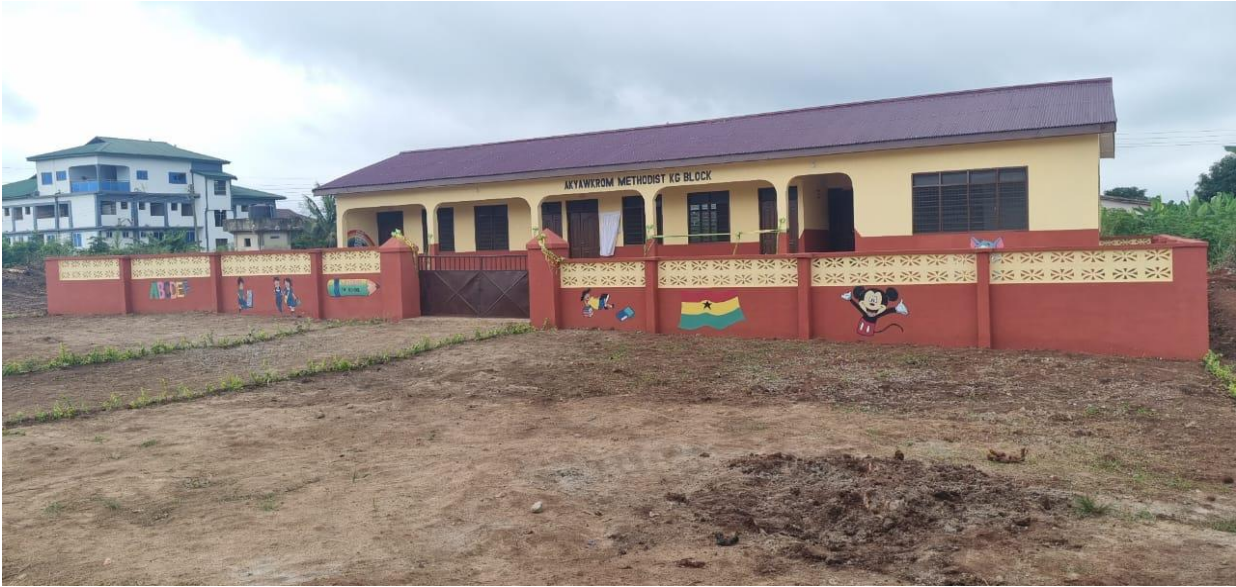
Completed 1No. 2-Unit KG Block with store, office, kitchen, washrooms and fence wall, in use at Akyawkrom
