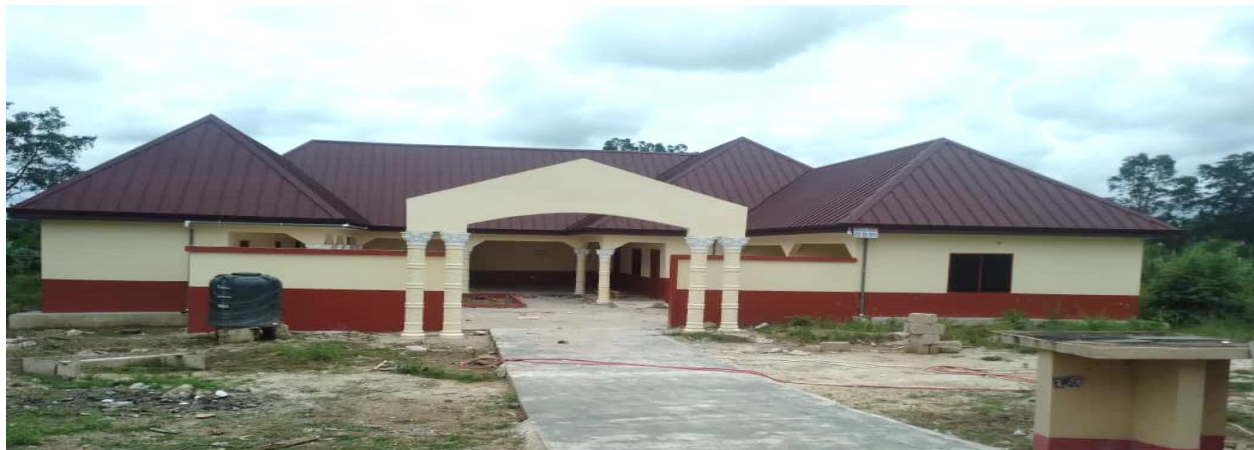
CONSTRUCTED 1NO. 3-UNIT WARD WITH ANCILLARY FACILITIES AND SUPPLY OF HT03 MANUAL BED AT NKASEIM. FUND SOURCE: DACF-RFG
