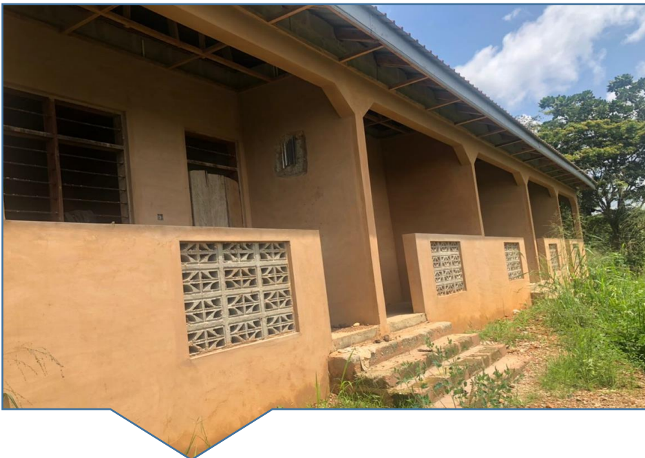
Construction of a Staff Quarters at Asankrangwa
