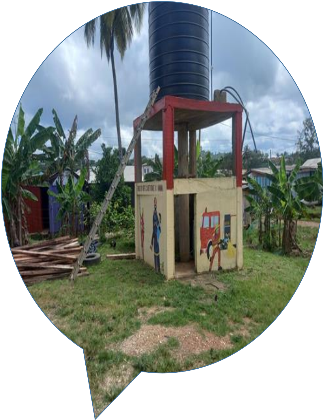
Completion of Mechanised borehole with polytank at Asankrangwa Fire Station.
