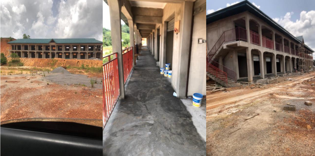
15. Construction of Market at Huni Valley
