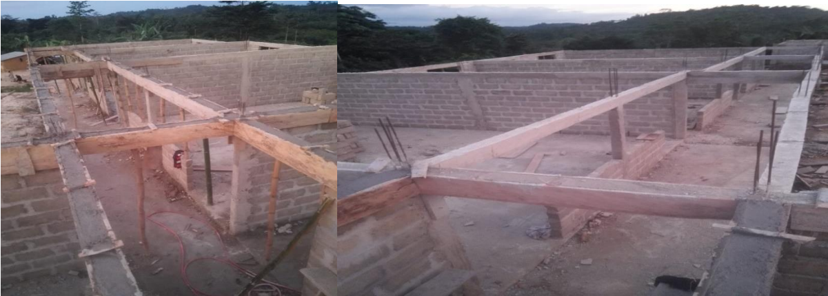
14. Construction 1No 6-unit classroom block at Broni Nkwanta
