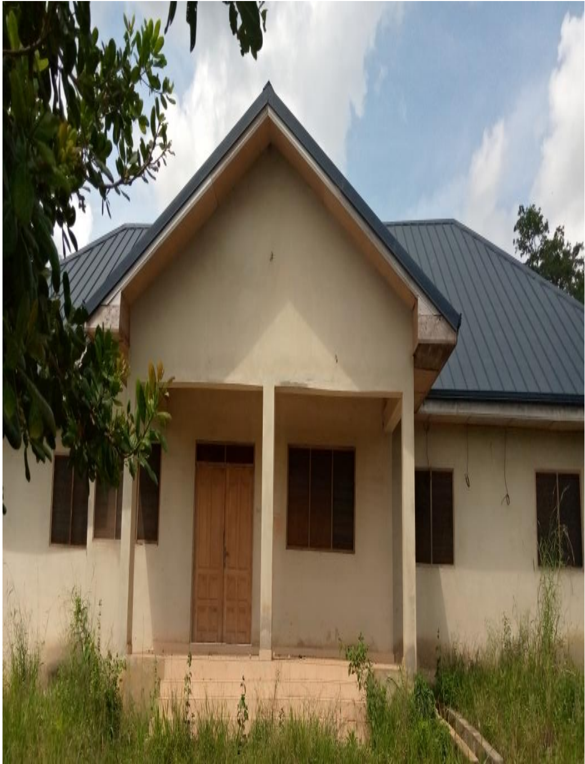
Constructed 1No. Police station with 4 Unit quarters
