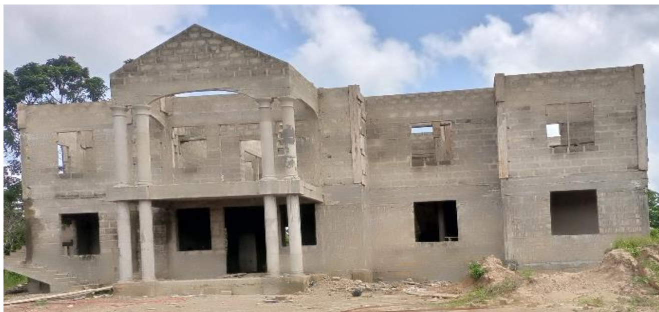
Constructed 1No. 2 unit KG block at Comey (Enchi) complex at Ajakaa
