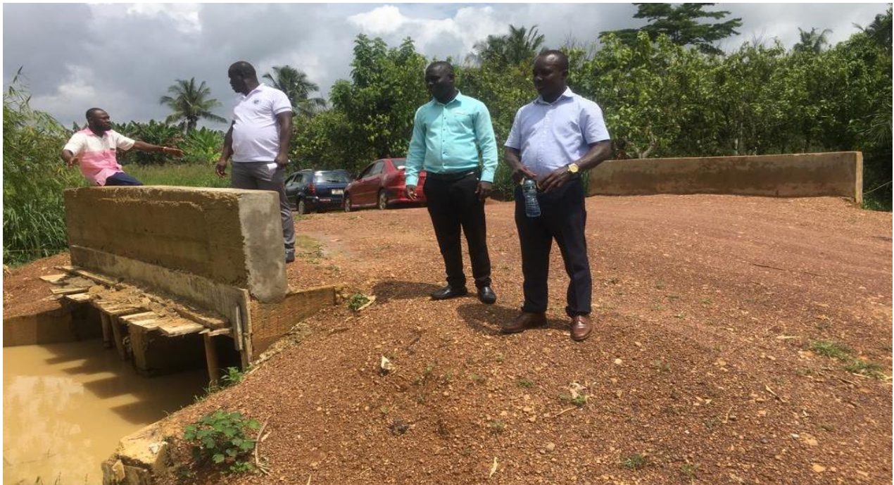
Constructed 1No 1.5m Box culvert on Jensuu Kwasiakrom Road
