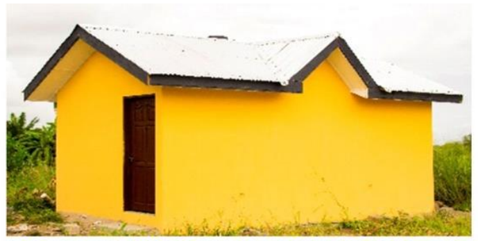
Constructed 1No 6-seater WC at Mafi-Kumase Senior High Technical School
