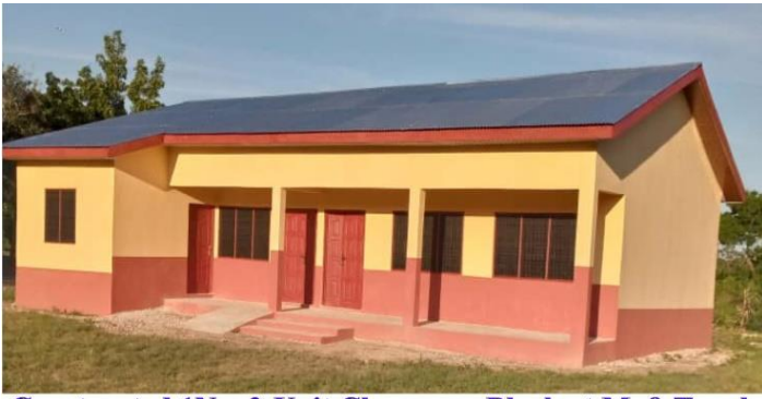
Constructed 1No. 2-Unit Classroom Block at Mafi-Tsawla
