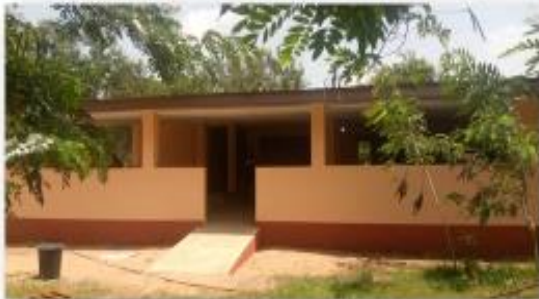
CONSTRUCTED OPD AT KPOTAME CHPS COMPOUND
