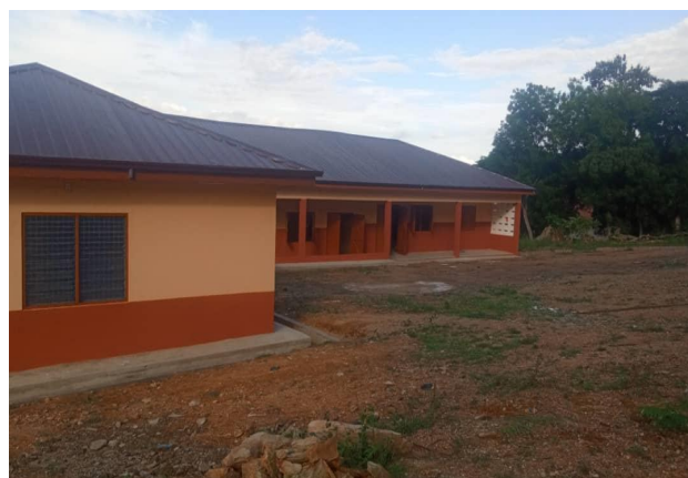
3 Unit Classroom Block at Kpalime Dugah
