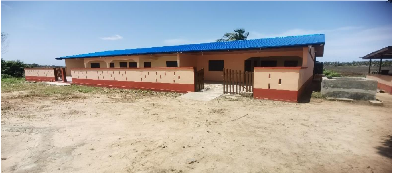
Construction and completion of 1No. CHPS Compound and nurses quarter at Akame
