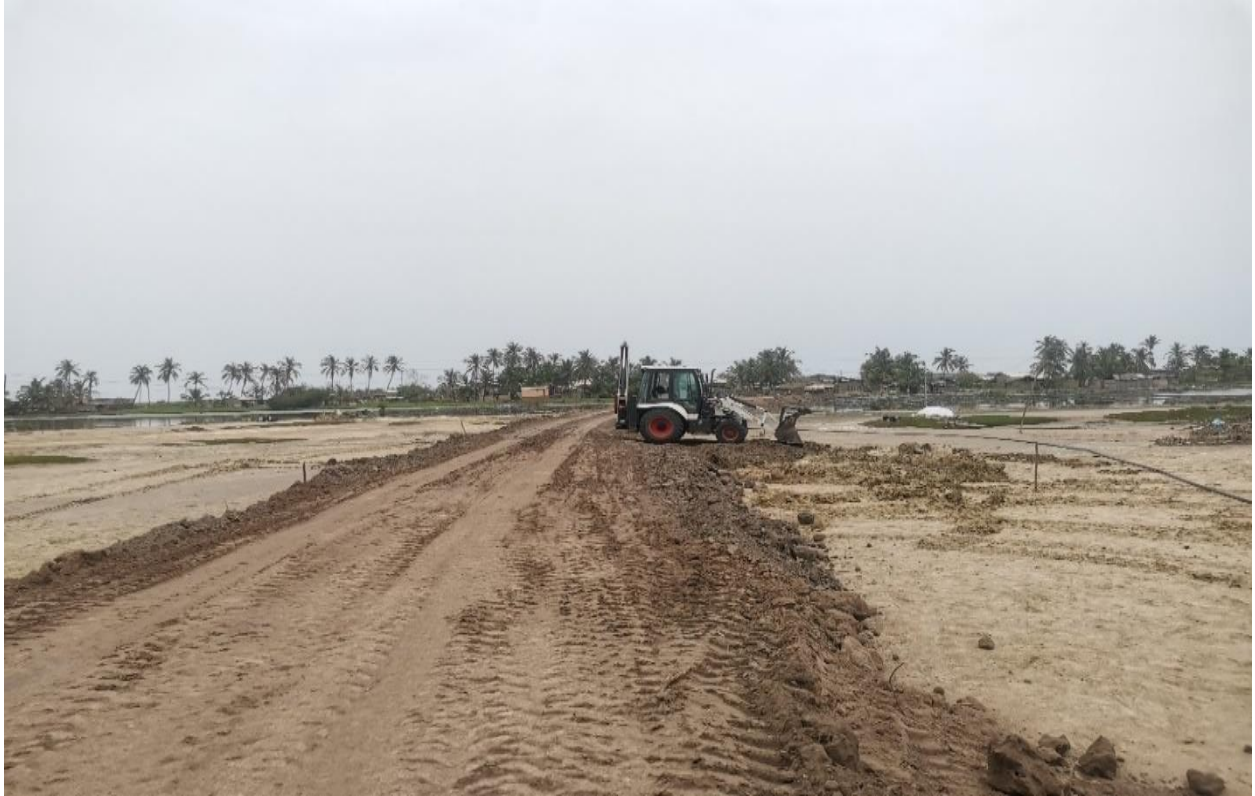
Construction of road to Salakope resettlement community for Tidal wave victims.
