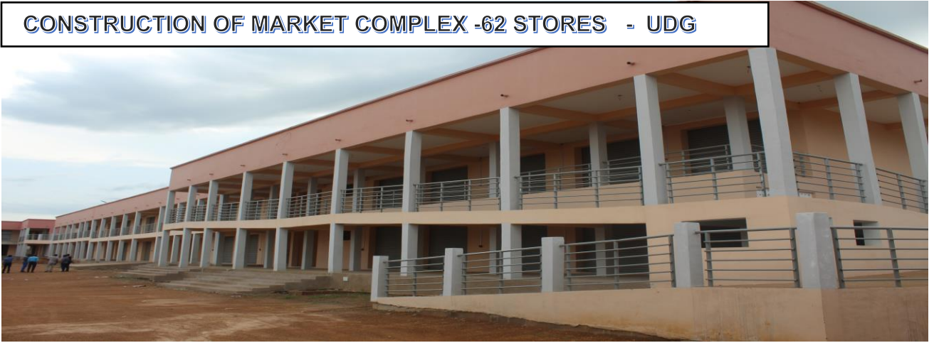
CONSTRUCTION OF MARKET STALLS - UDG
