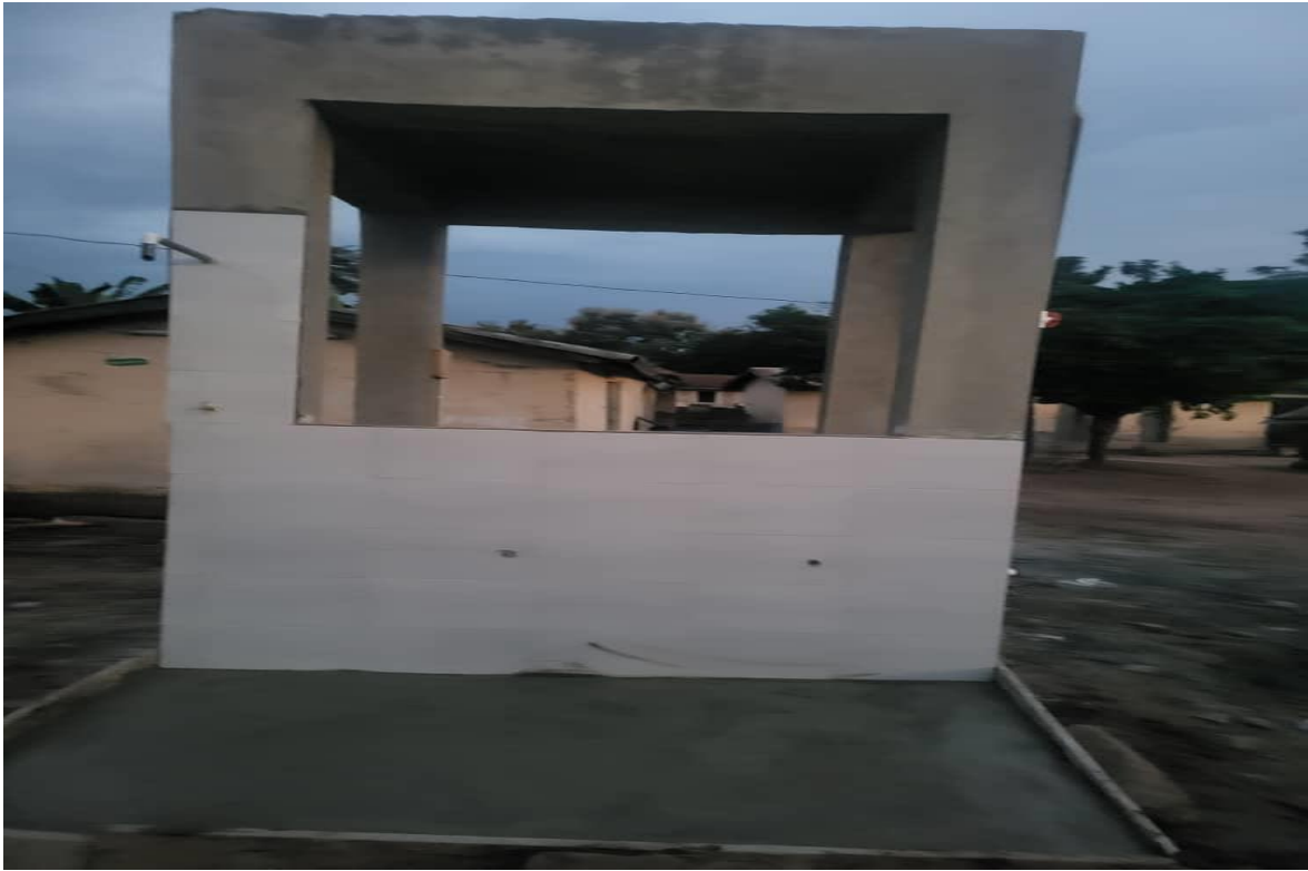
Construction and mechanization of borehole at Have
