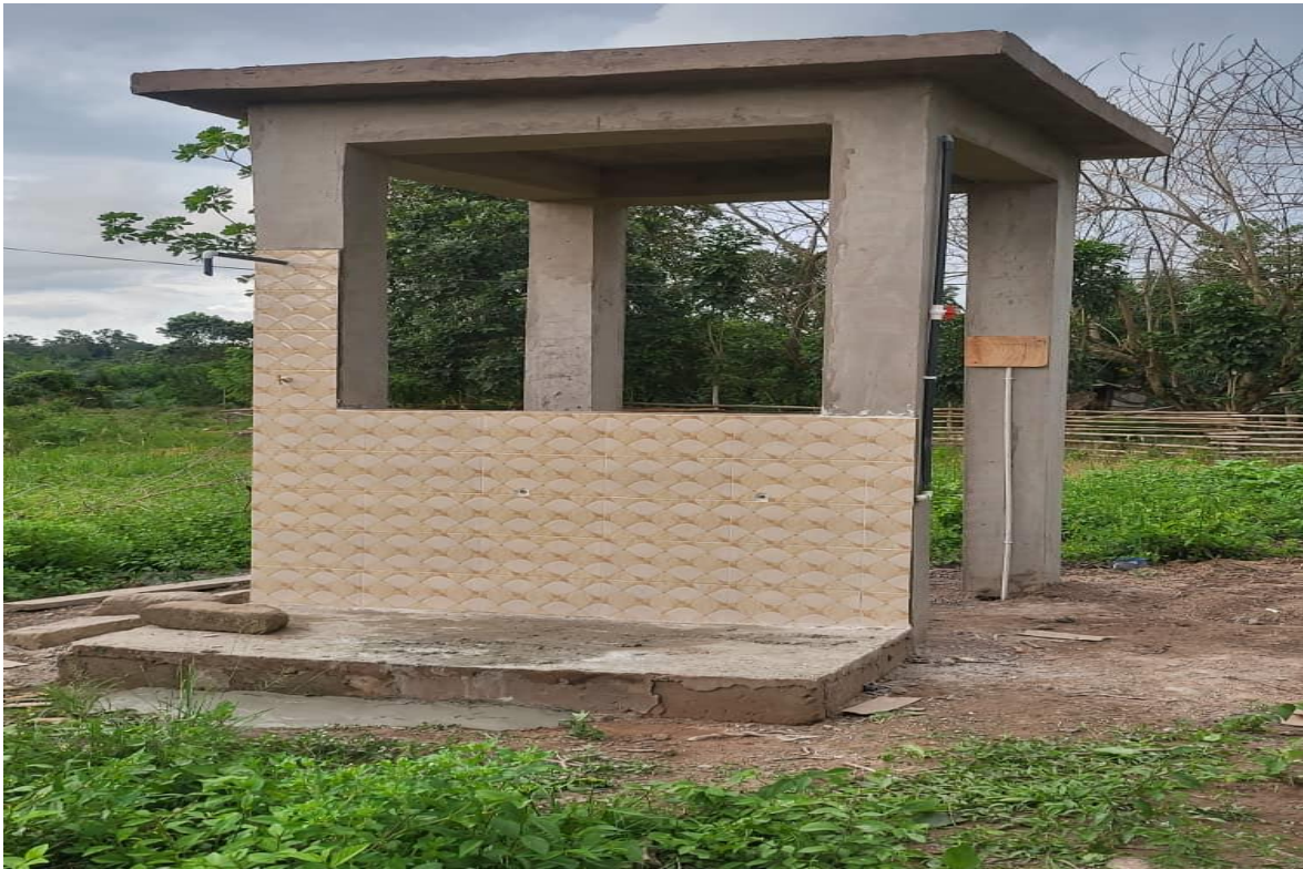
Construction and mechanization of borehole at Nyagbo Bethel
