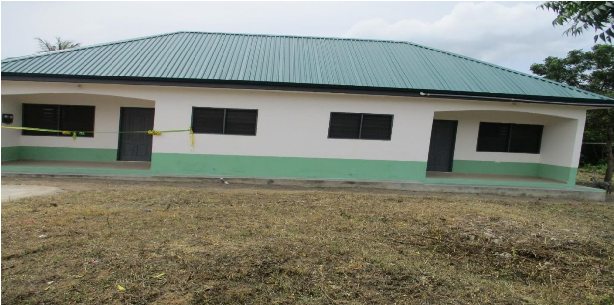
Completed and Commissioned Hlihava Nurses Quarters
