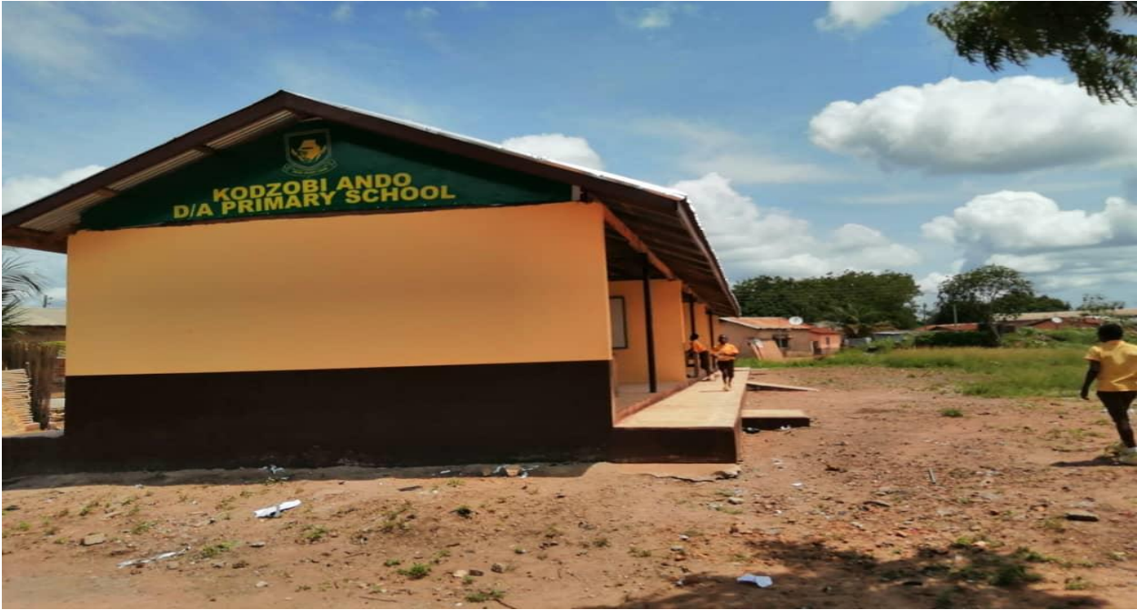
Completed and Handed over Kodzobi D/A Basic School Pavilion to GES
