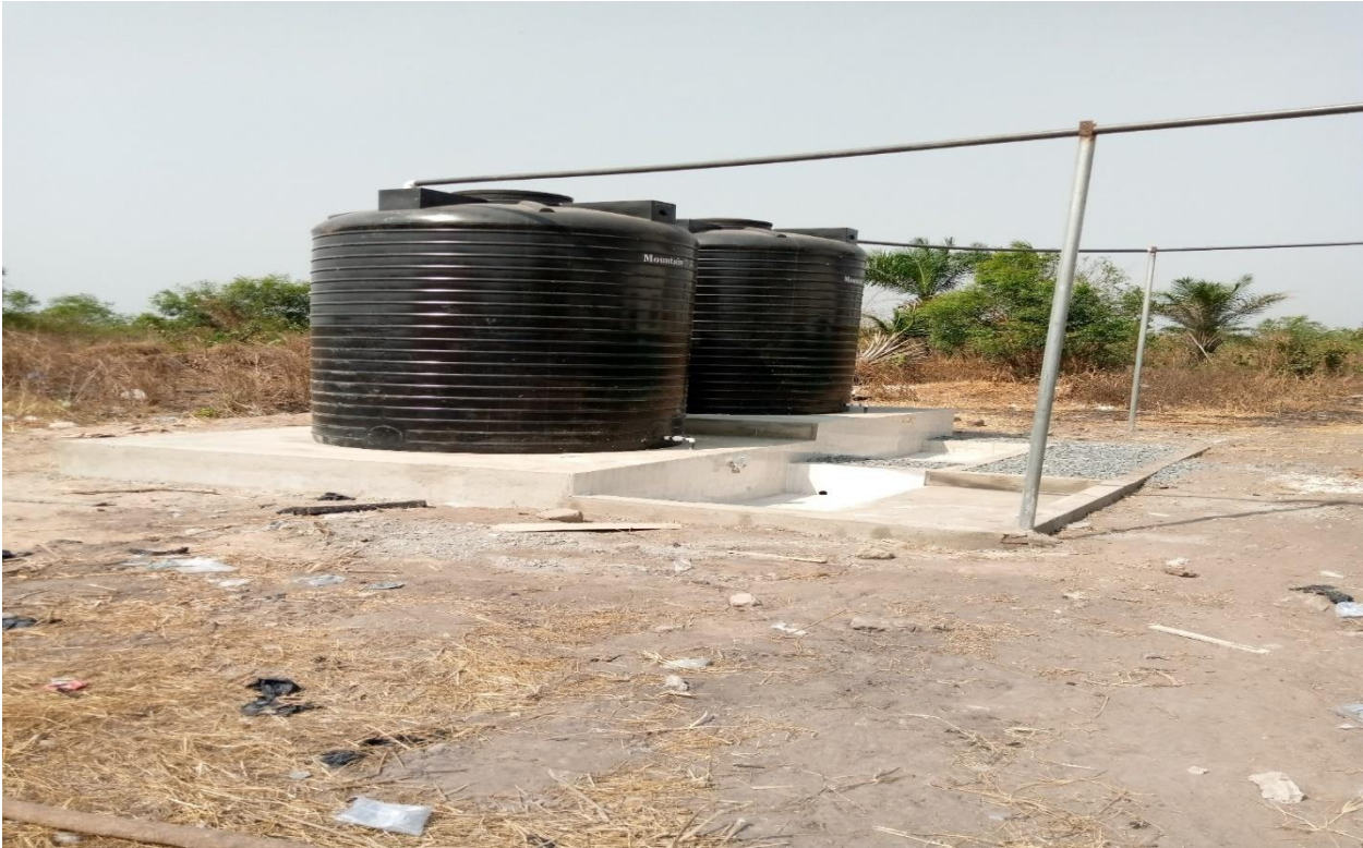
Constructed Waya Animal Market Water Storage Facility
