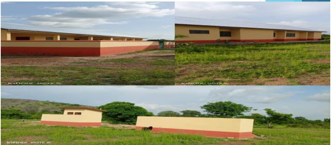
1No. CHPS Compound Constructed at Ombo-Kahaa
