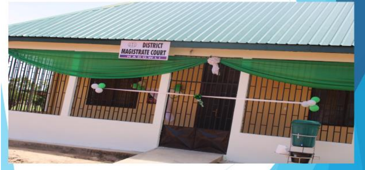
Nadowli Magistrate Court completed.
