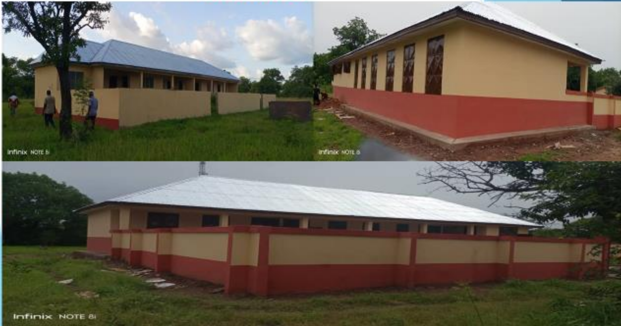
KG Block with Gender Ancillary Facilities Constructed at Changu.
