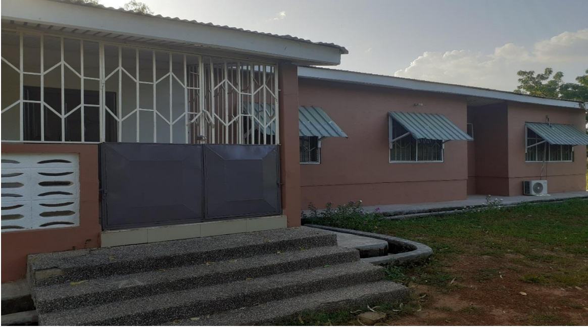
Picture of renovated Municipal Director Bungalow
