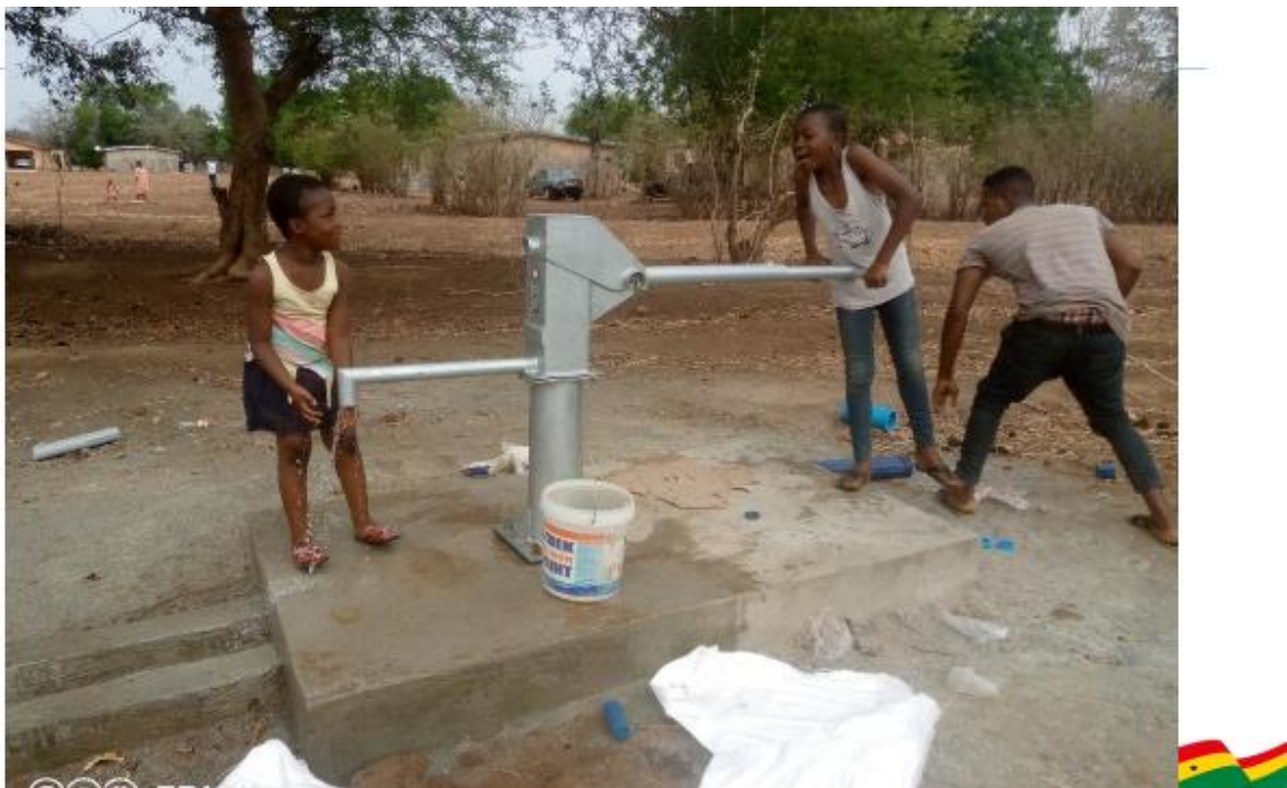
Figure 3: ON OF THE 13 BOREHOLES
