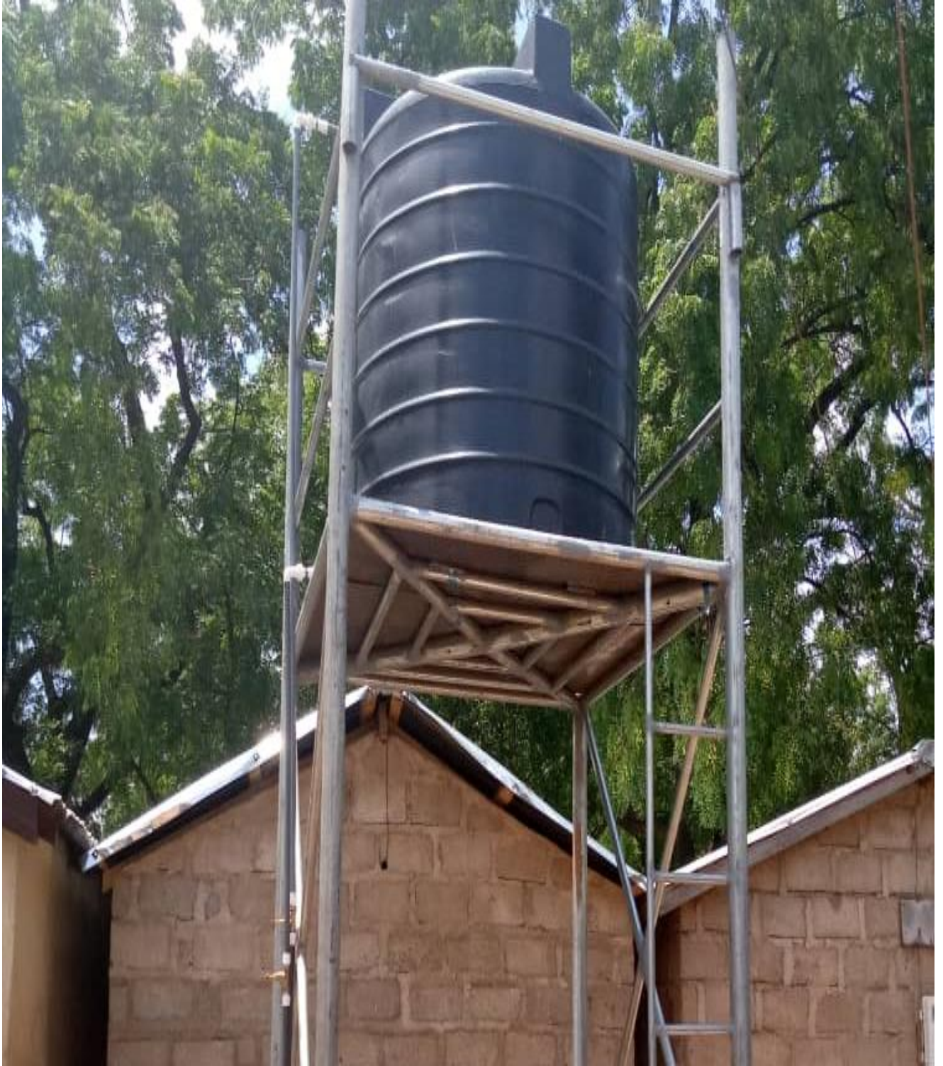
EXTENSION OF WATER WITH POLYTANK -RESERVOIRS TO PAGA MARKET
