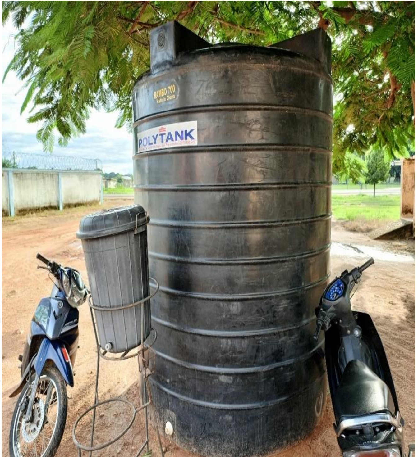
Drilling and Installation of Mechanised water systems at animal Kraal, Police Station and Fire Service
