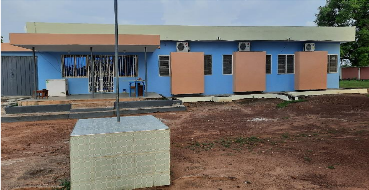
Renovated 1no. MCE's Residence at Suwarinsa (DACF)
