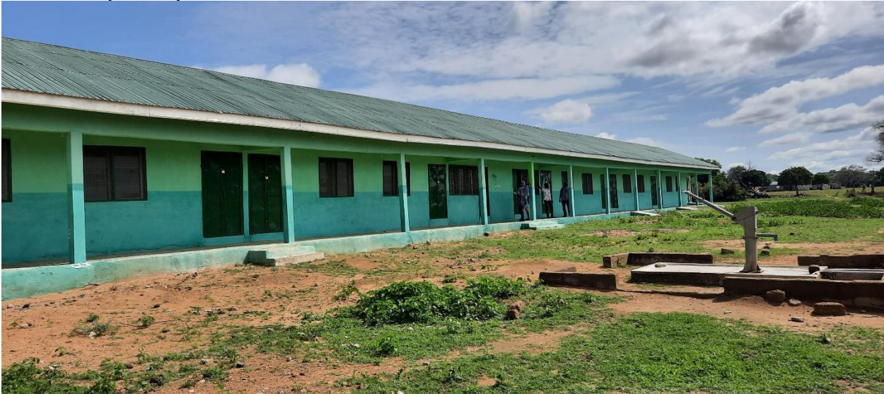
Constructed Chuchuliga SHS Classroom Block with Ancillary Facilities at Nawaasa (MPCF)
