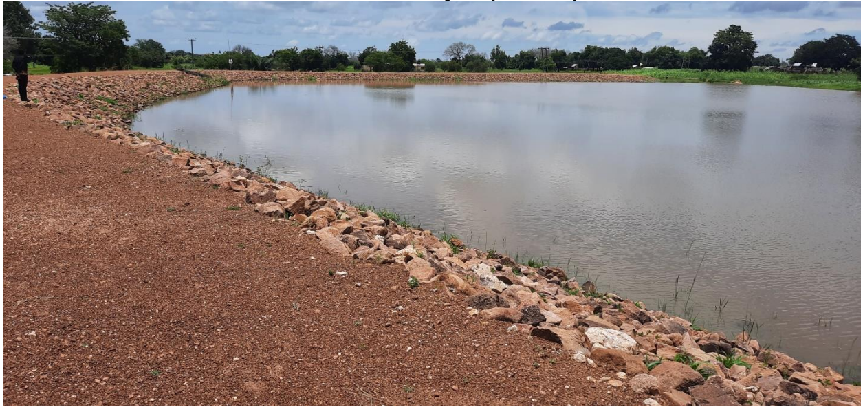
Rehabilitated 1no. Small Earth Dam at Kalijisa (GPSNP)
