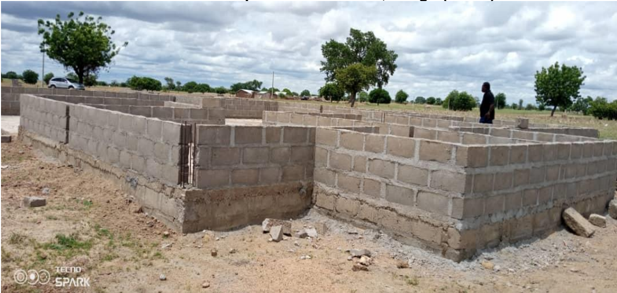
Construction of 1No. CHPS Compound at Yimonsa, Wiaga (DACF)
