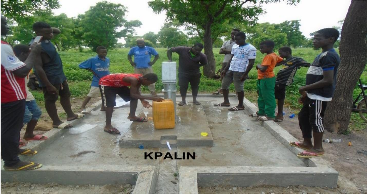
Figure 2. Drilling and Construction of Boreholes
