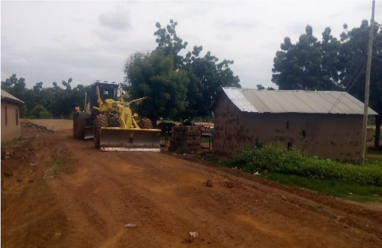
Figure 3. Opening up of Yogu - Wawani Feeder Road (3.5Km)
