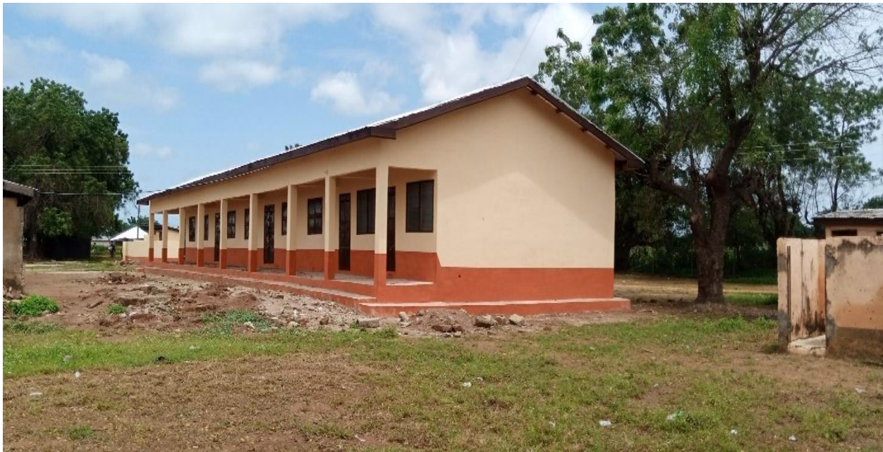
Figure 1. Construction of 1 No. 3 Unit Classroom block with ancillary facilities at Diare
