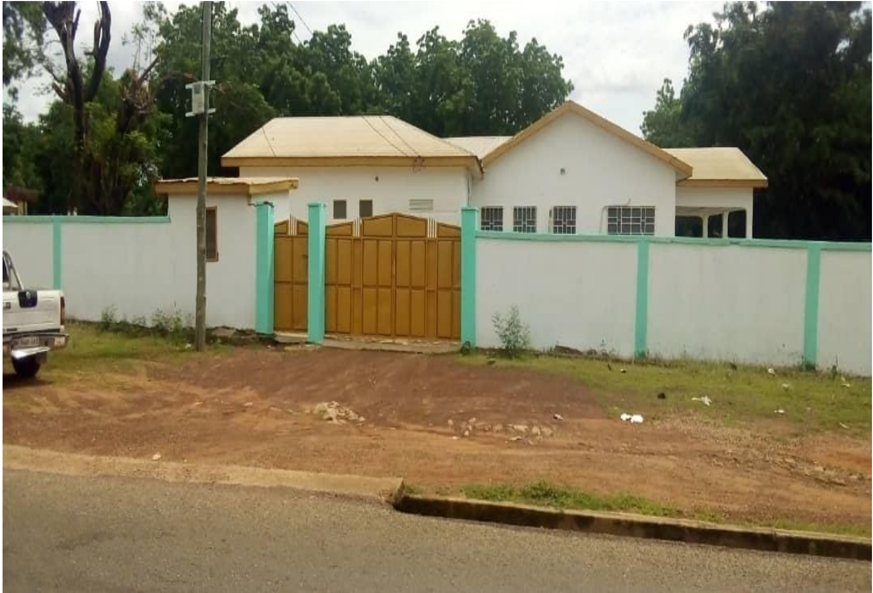
ABOVE: Rehabilitation of Municipal Chief Executive's residence
