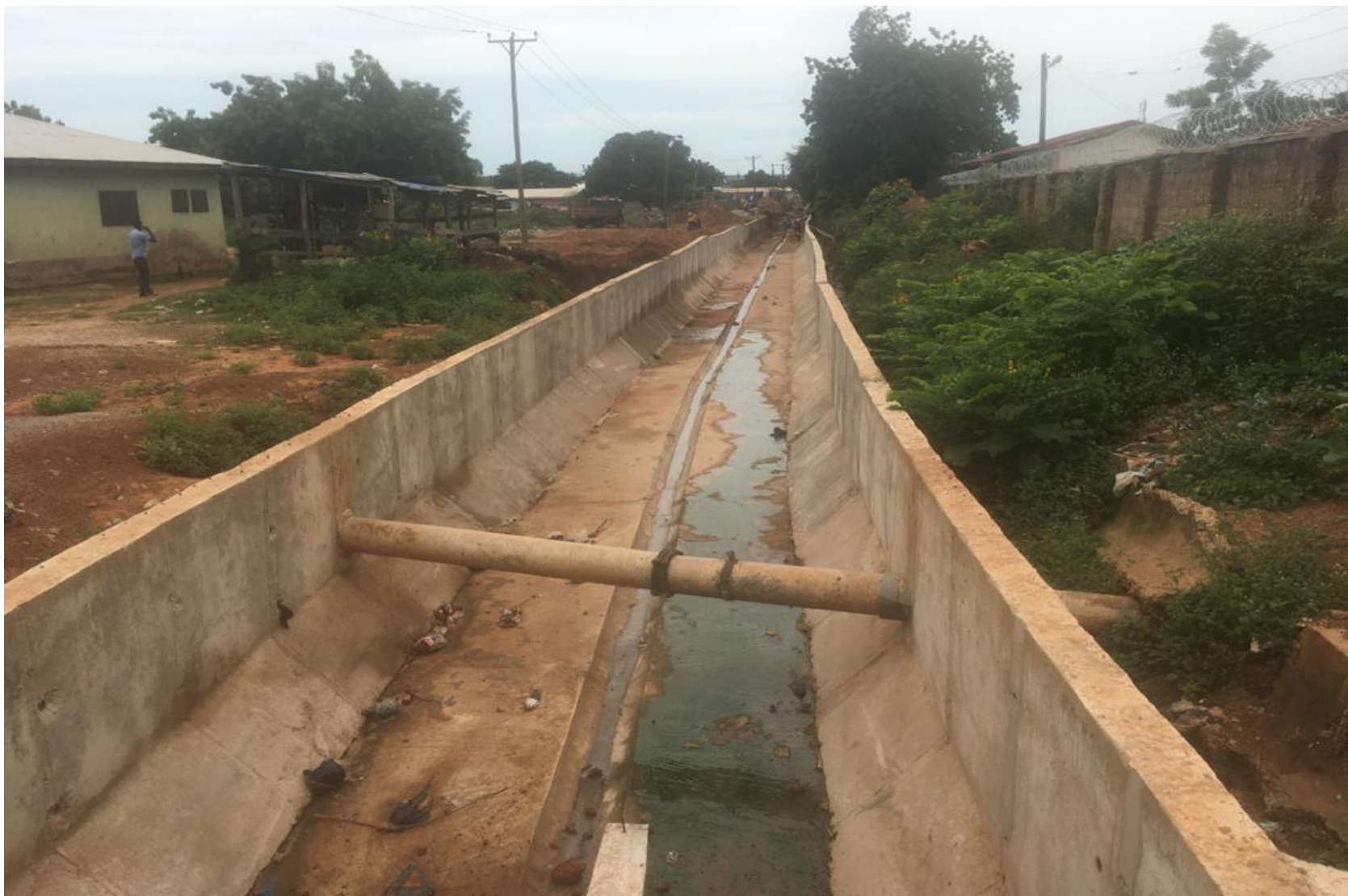
ABOVE: Completion of 800M Storm Drain at Ward-K.
