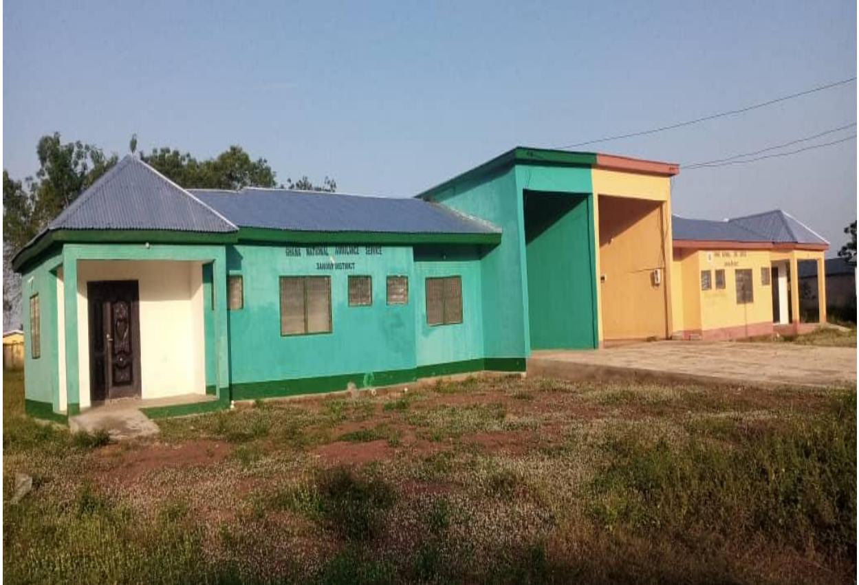
Newly Constructed Fire and Ambulance Stations
